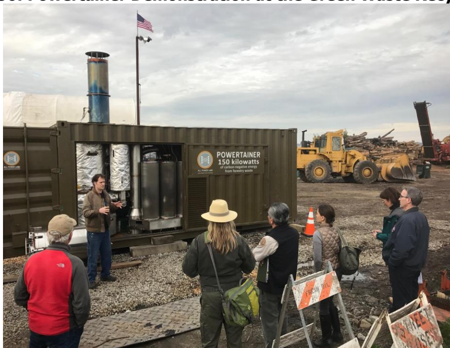
Figure 36: Powertainer Demonstration at the Green Waste Recycle Yard
