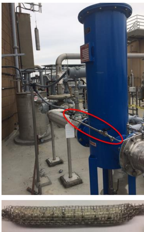
Installation of slipstream testing apparatus (top); sample of composite metal-organic framework pellets for exposure testing (bottom).
