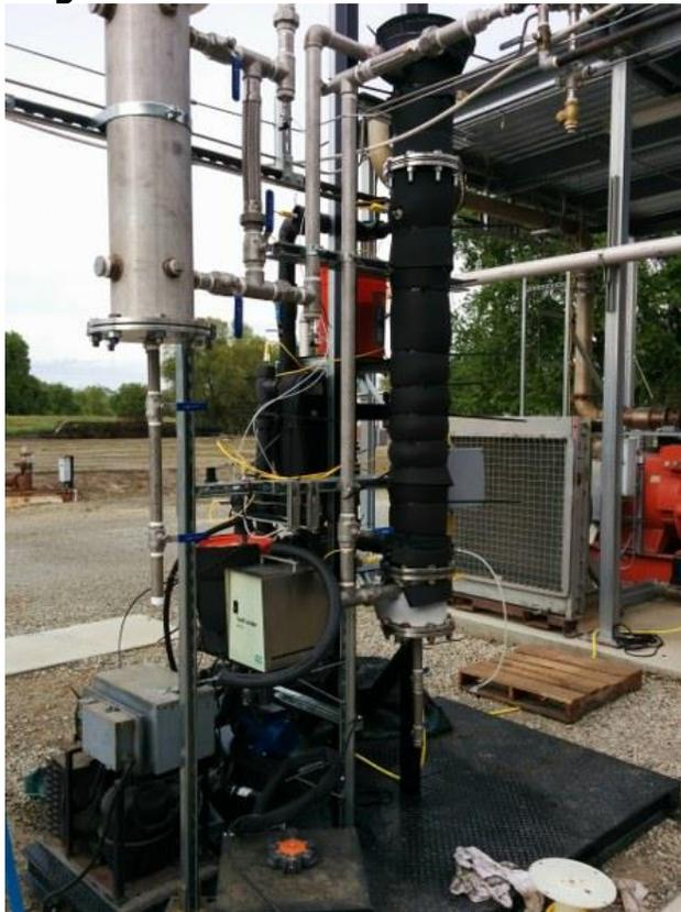
Photograph of installed chilled biodiesel scrubber (right vessel) with piping and chilling equipment. Producer gas enters near the bottom of the chilled scrubber. On the left side, an adsorbent vessel is shown, used for moisture removal before the piston compressor. Gas sampling ports are available after each unit for the analysis of gas, sulfur, and tar compounds.
