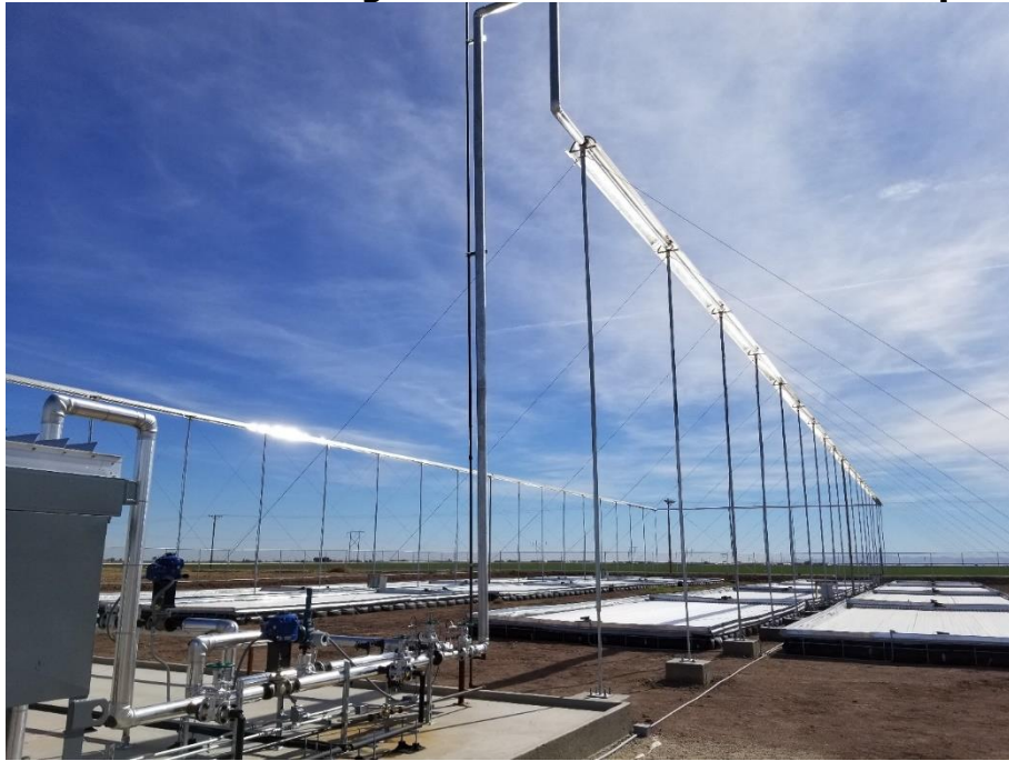
Figure 12: Concentrating Solar Power Construction Complete
