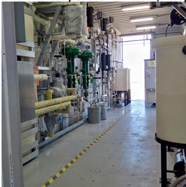
Figure 14: Container after Completion of Fabrication, Ready for Operations
