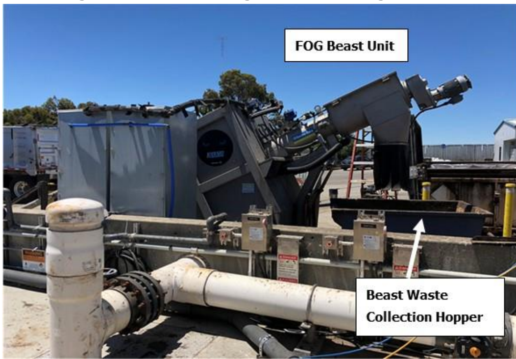
Figure 6: FOG Receiving Station Showing the Beast
