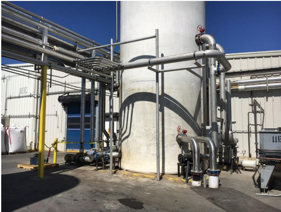
Figure 11: Existing Glycol Tank Modified to Receive Chilled Glycol from the ThermoSorber
