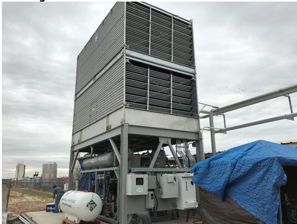
Figure 12: Cooling Tower Installed Above ThermoSorber for Warm-Water Loop
