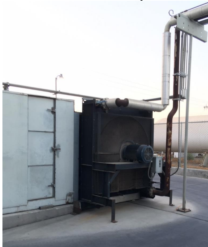
Figure 14: Repurposed Radiator Used to Transfer Heat from the Hot-Water Loop to the Procream Dryer
