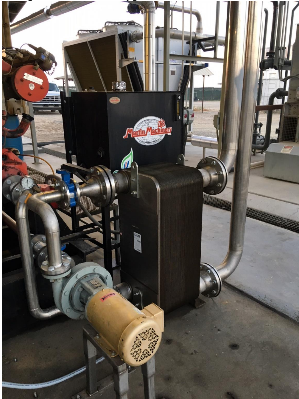
Figure 8: Oil Coolers Upgraded for Each 800 KW Genset
