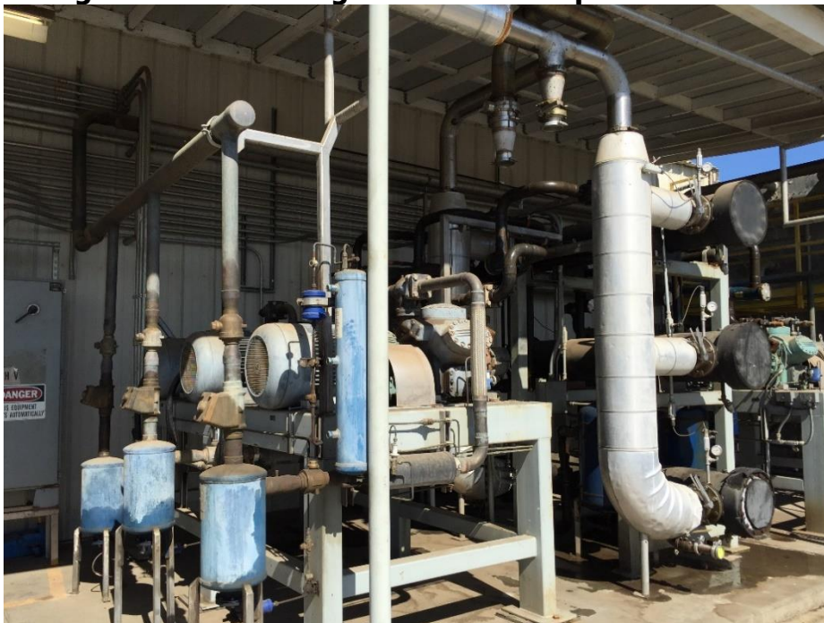
Figure 3: Preexisting Chillers at Joseph Gallo Farms
