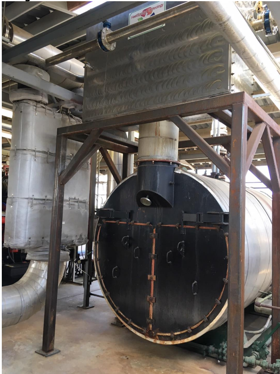
Figure 9: Exhaust Economizer Installed Above Boiler
