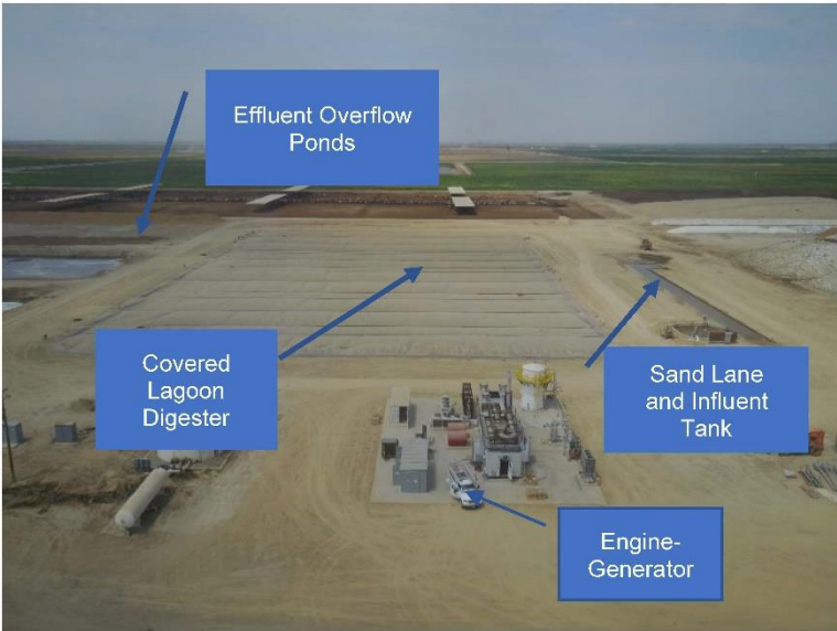
Figure 4: ABEC #3 Overview of Digester System
