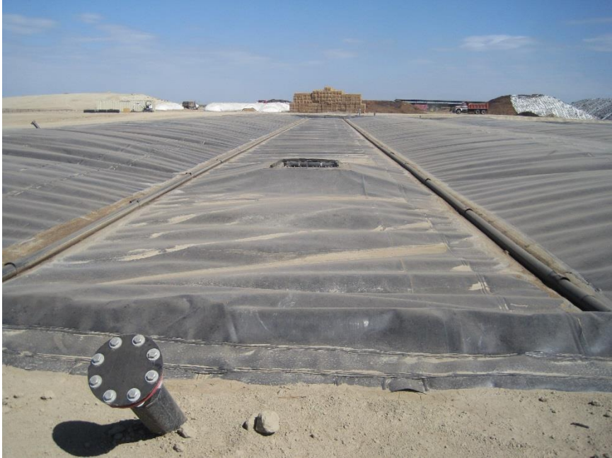
Figure 3: ABEC #3 Digester Cover Installation
