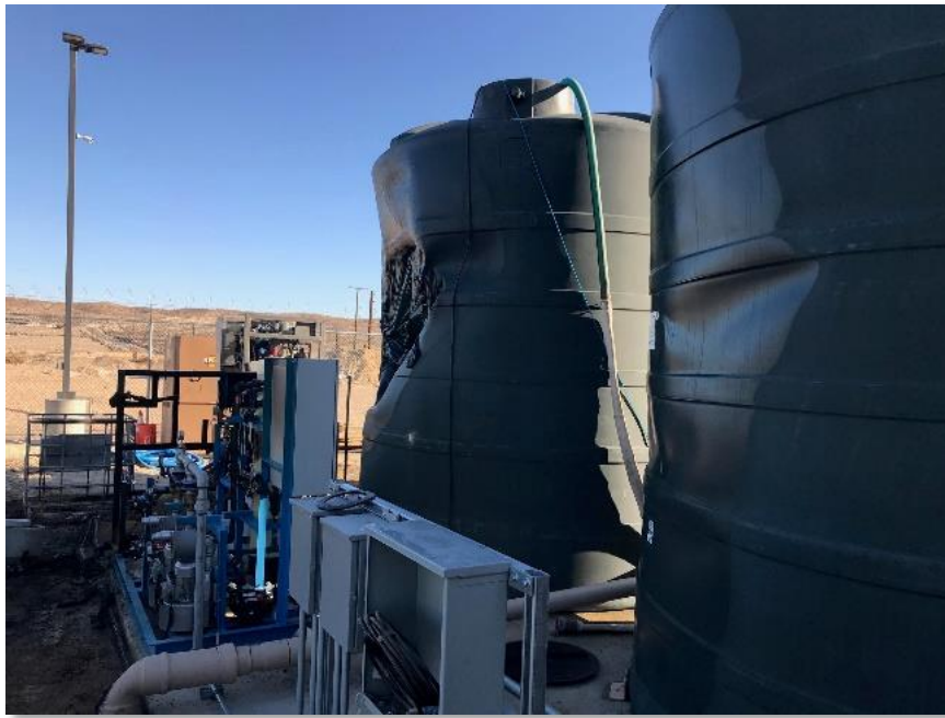
Figure 6: Damaged View of Storage Tanks and Post-Treatment Process
