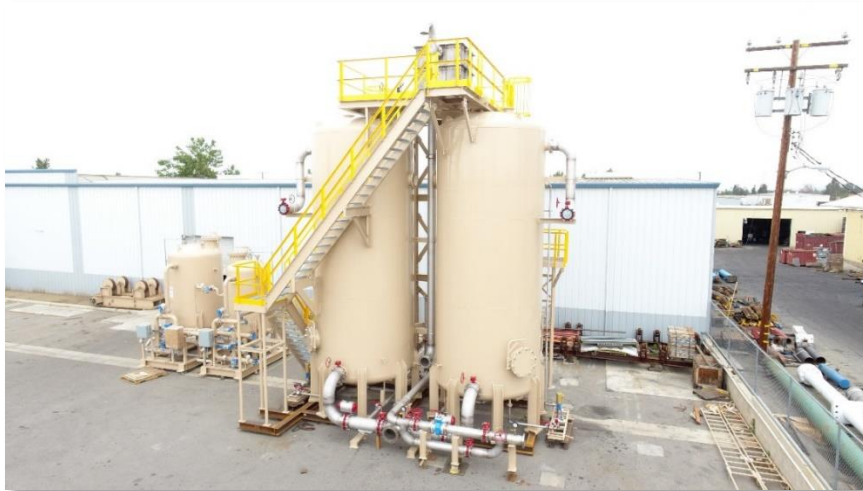
Figure 4: Fabricated Biofiltration System Vessel and Connection Devices
