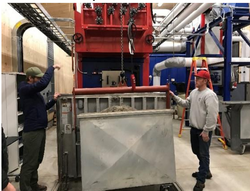
Figure 9: High Sierra Community Energy Development Corporation Owner Trains Plumas County Facilities Staff on Ash Bin Removal
