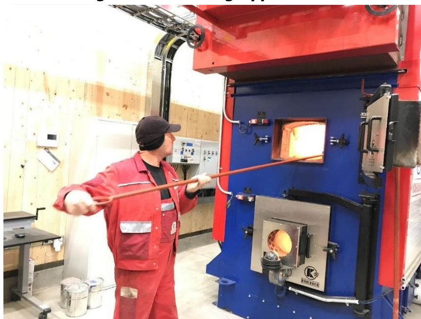
A boiler technician demonstrates how to clean the upper furnace.
