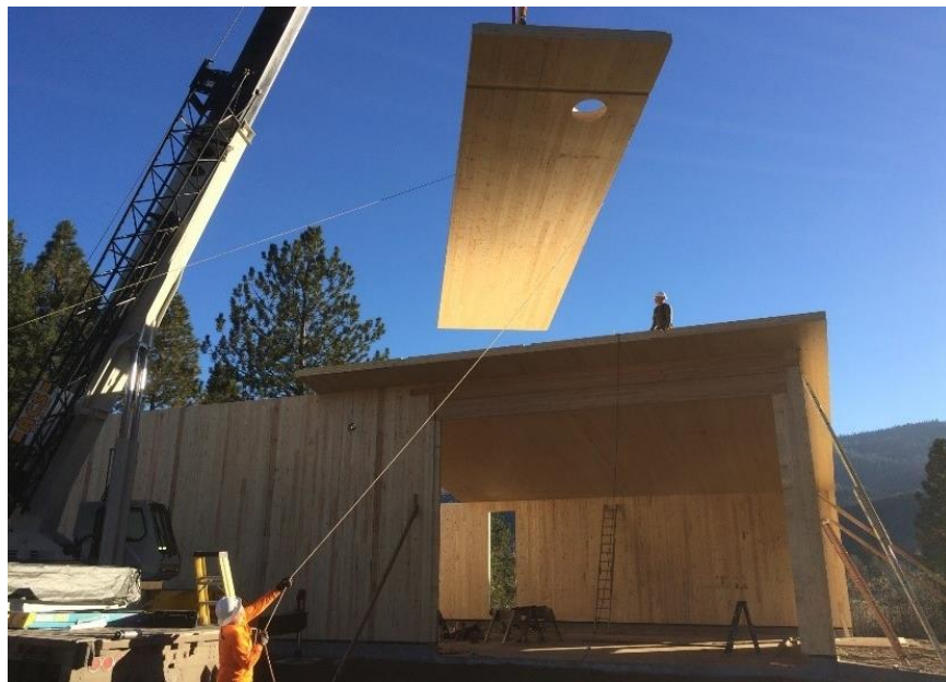
Figure 7: Construction of Cross-Laminated Timber Building
