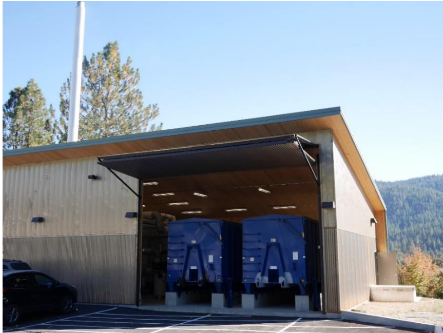
Figure 12: Wood Chip Storage Bins Inside Boiler Building
