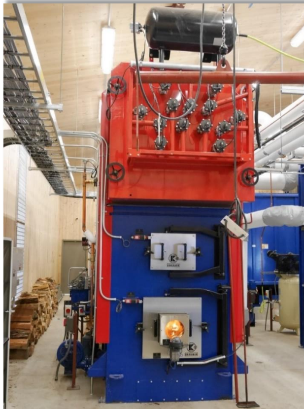
Figure 3: Plumas Health and Human Services Center Biomass Boiler Fired Up
