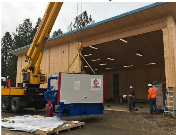
Figure 10: Kohlbach Furnace Being Unloaded and Installed
