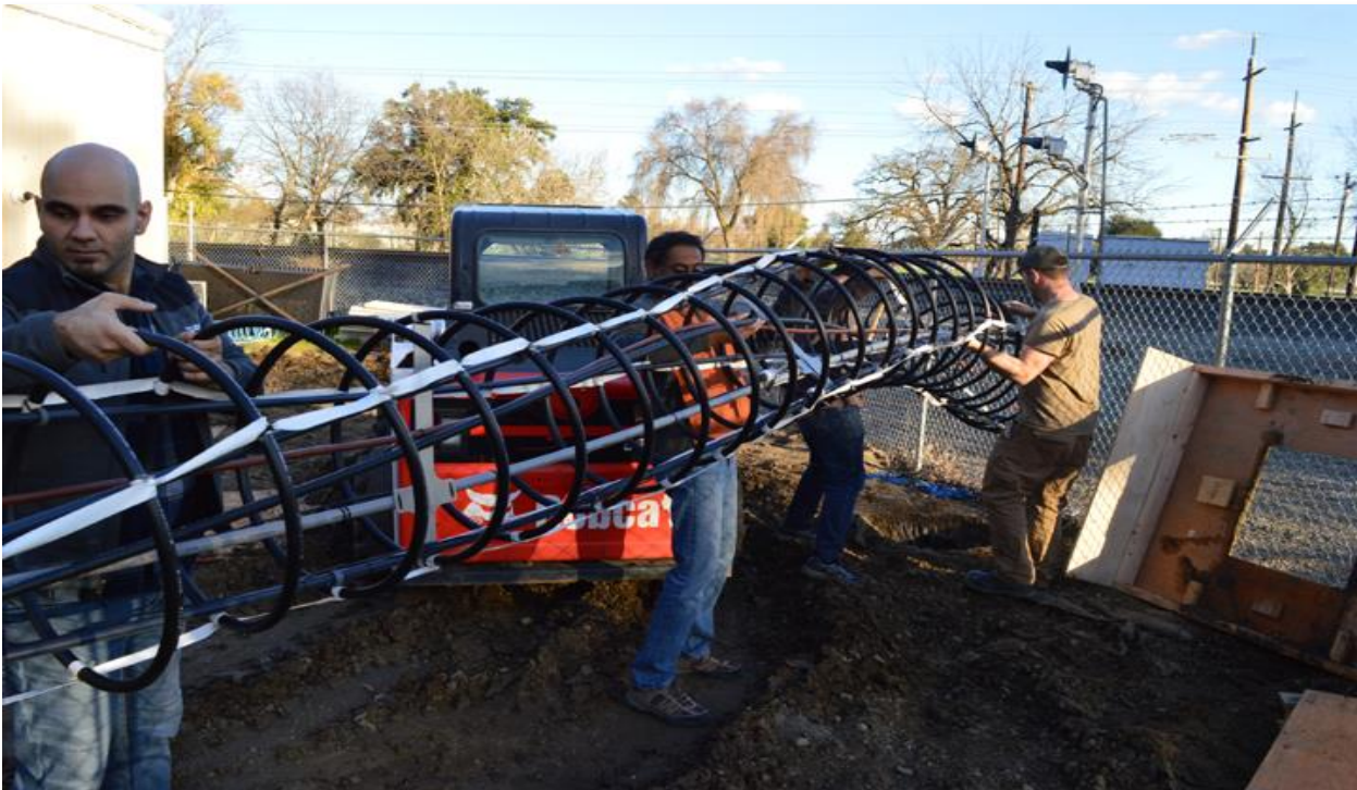
Figure 2: Installation of Ground Heat Exchanger into Bore
