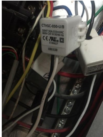
Figure 6: Electric Meter Current Transducers (CTs)
