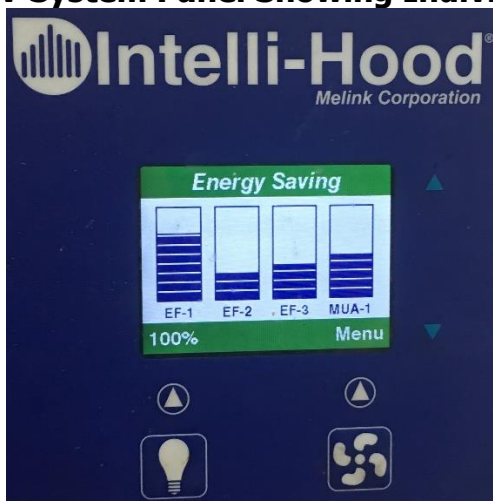
Figure 278 DCKV System Panel Showing Individual Fan Speeds
