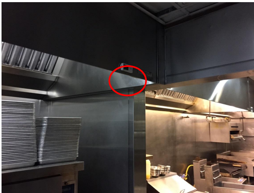
Figure 223: Prep Line Ambient Temperature Measurement Near Convection Oven
