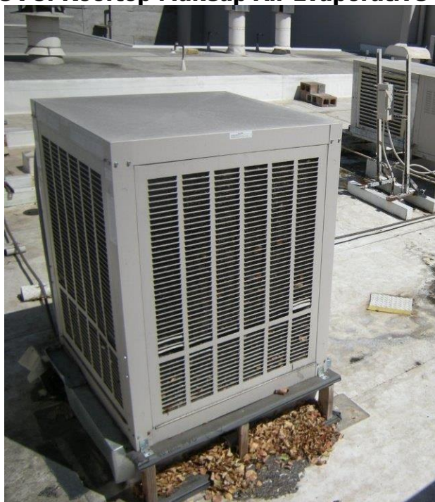
Figure 78: Rooftop Makeup Air Evaporative Cooler
