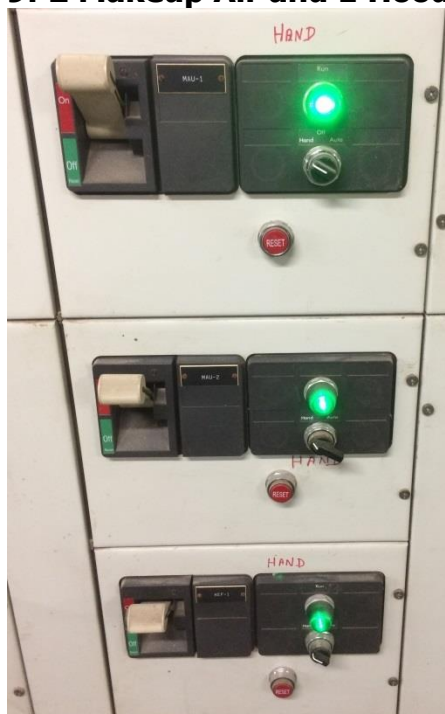
Figure 79: 2 Makeup Air and 1 Hood Breaker
