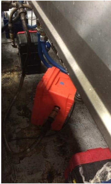
Figure 4: Enclosed Gas Meters Installed at Doubletree Hotel
