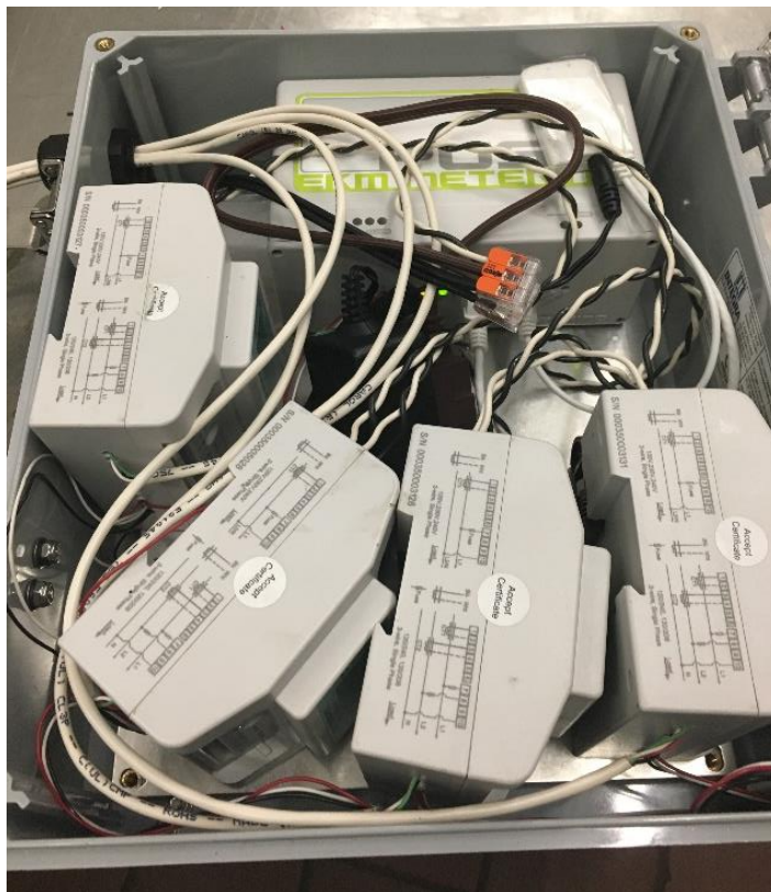
Figure 280: EIS Data Collection Hardware with 3 Transmitters in a Central Location
