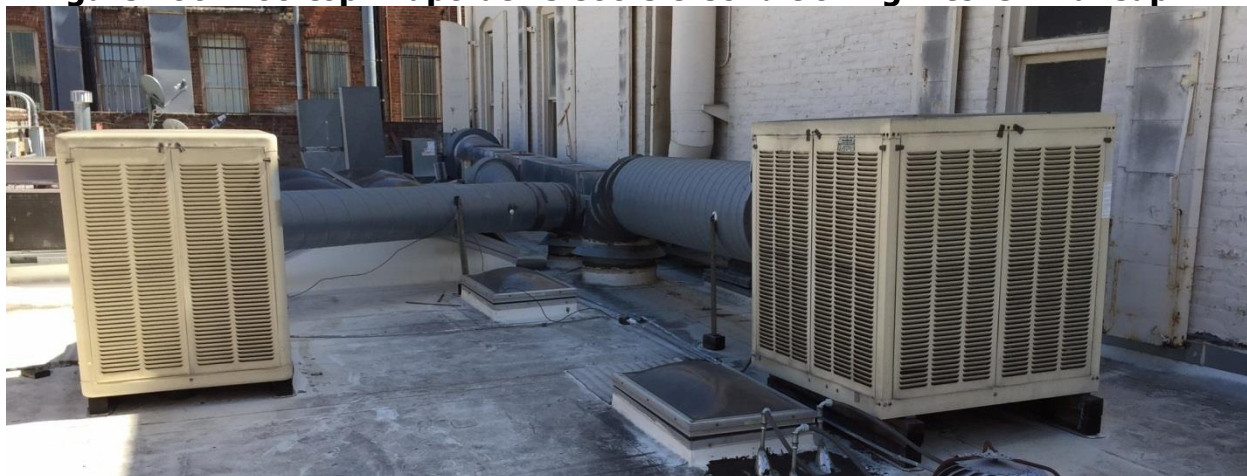
Figure 206: Rooftop Evaporative Coolers Conditioning Kitchen Makeup Air
