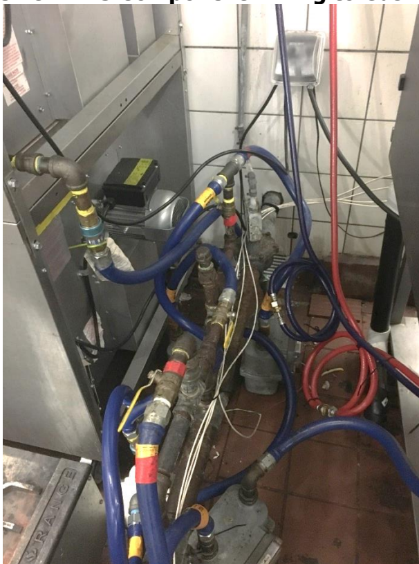
Figure 281: EIS Component Wiring to Gas Meters
