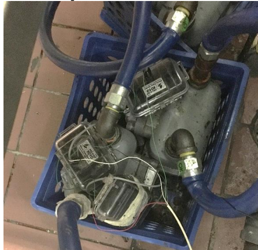
Figure 282: EIS System Connections at Gas Meters
