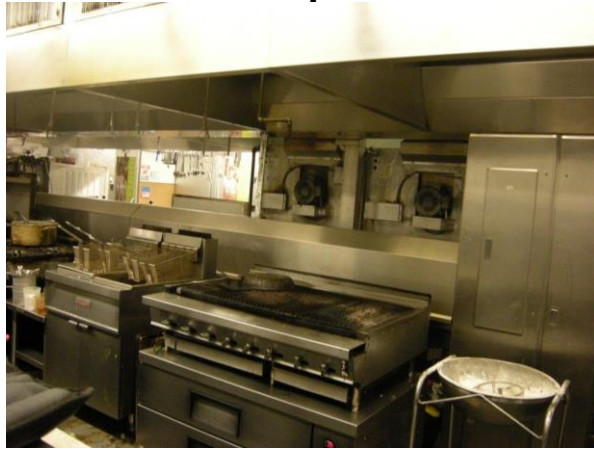
Figure 75: Hood Section Separation Above the Broiler
