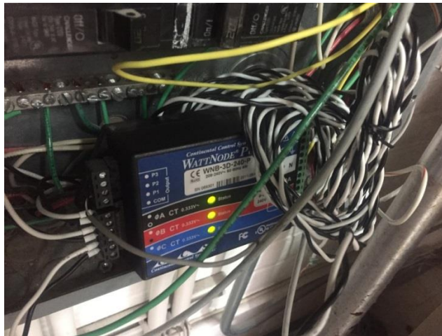
Figure 5: Electric Meter Inside Werewolf Panel: Ventilation Fan Monitoring
