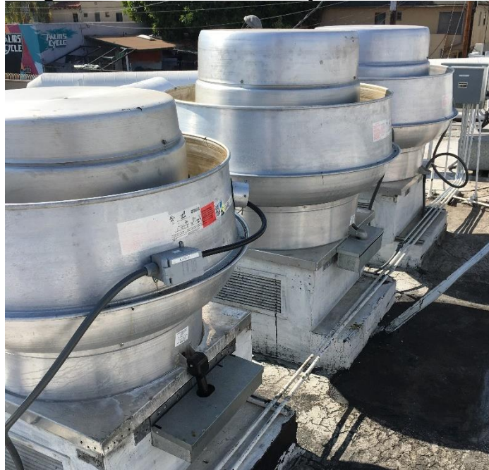
Figure 272: Three Rooftop Exhaust Fans
