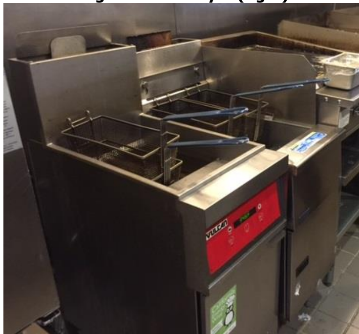
Figure 173: Replacement Super High-Efficient Fryer (left) and the Existing Budget High-Efficient Fryer (right)
