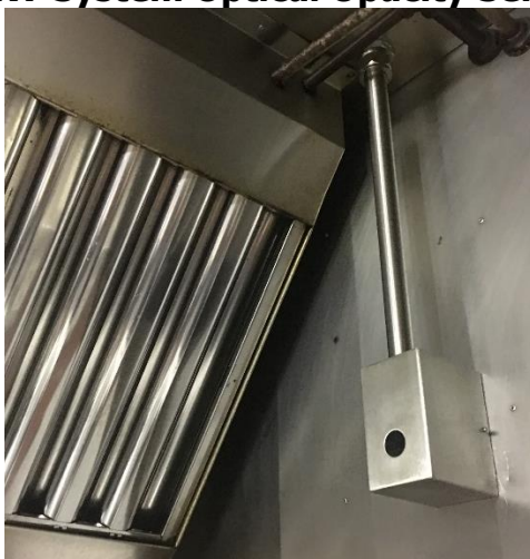
Figure 279: DCKV System Optical Opacity Sensor in the Hood
