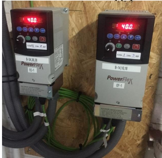
Figure 212: Exhaust and Supply Fan VFDs
