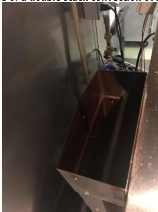
Figure 343: Flue of a double stack convection oven, 6-7 feet high
