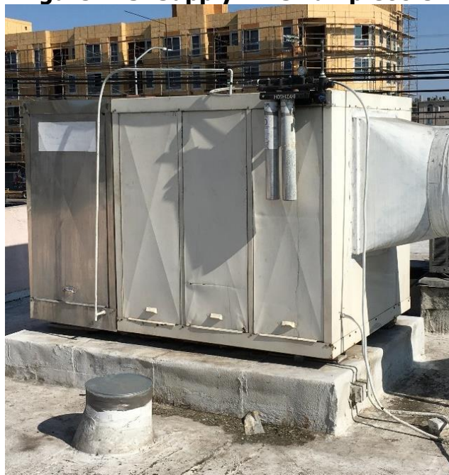
Figure 273: Supply Air Swamp Cooler
