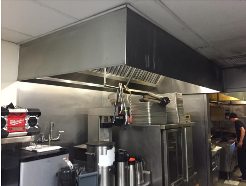
Figure 204: Prep Line Exhaust Hood with Convection Oven and Coffeemaker Underneath
