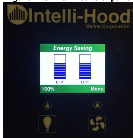
Figure 213: DCKV control panel
