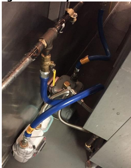
Figure 102: Fryer Gas Meters
