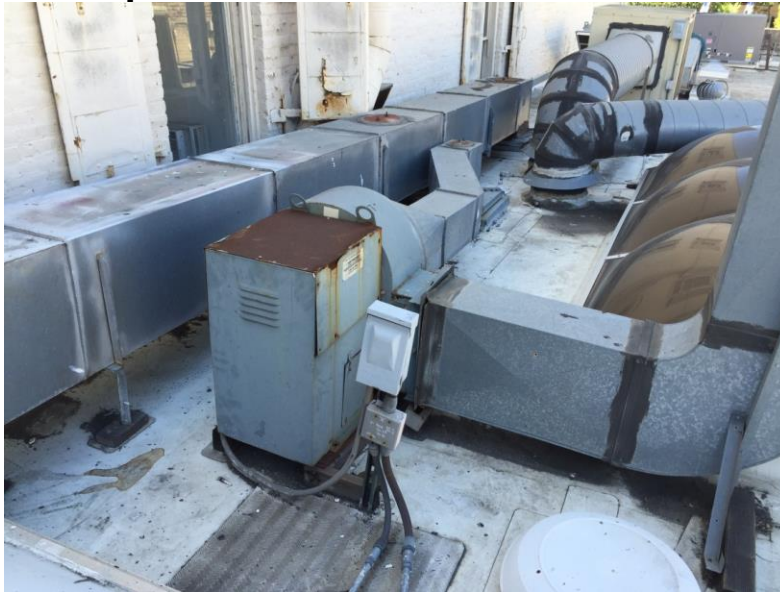
Figure 205: Prep Line Exhaust Fan on the Roof of the Restaurant
