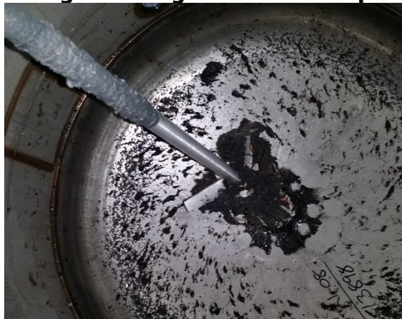
Figure 9: Digester Mixer Prop
