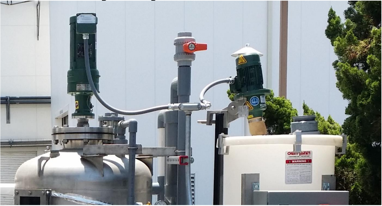
Figure 8: Digester and Feedtank Mixers
