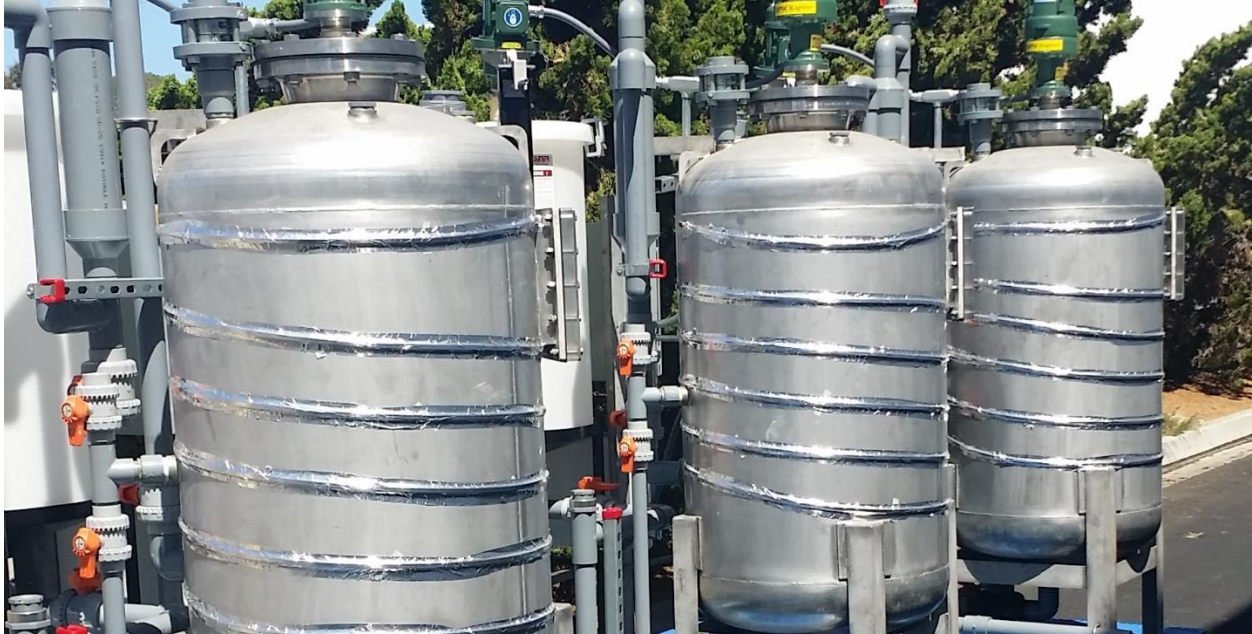
Figure 5: Heat Tracing Before Insulation
