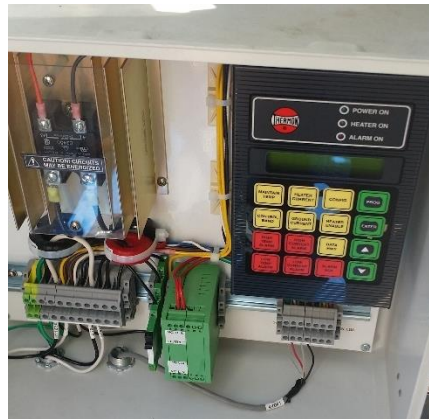
Figure 6: Heat Trace Control Panel
