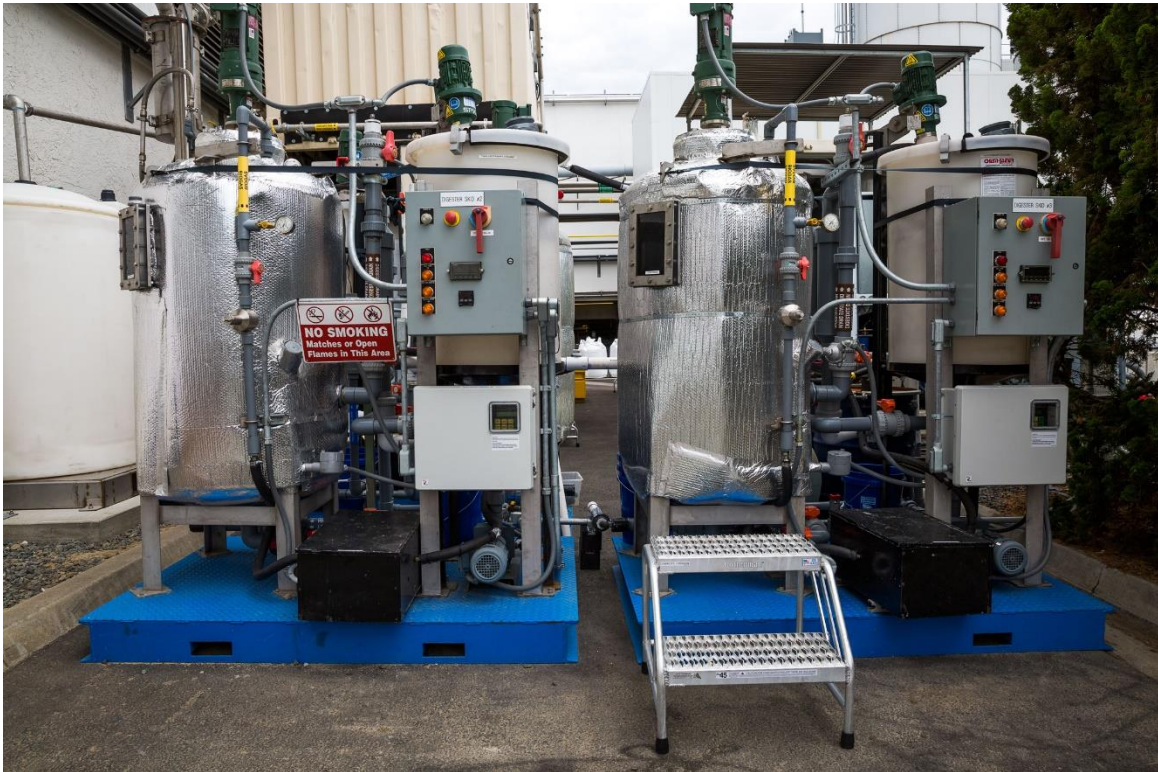
Figure 14: Back Side of Pilot Digesters with Electrical Control Panels and Heat Trace Controllers
