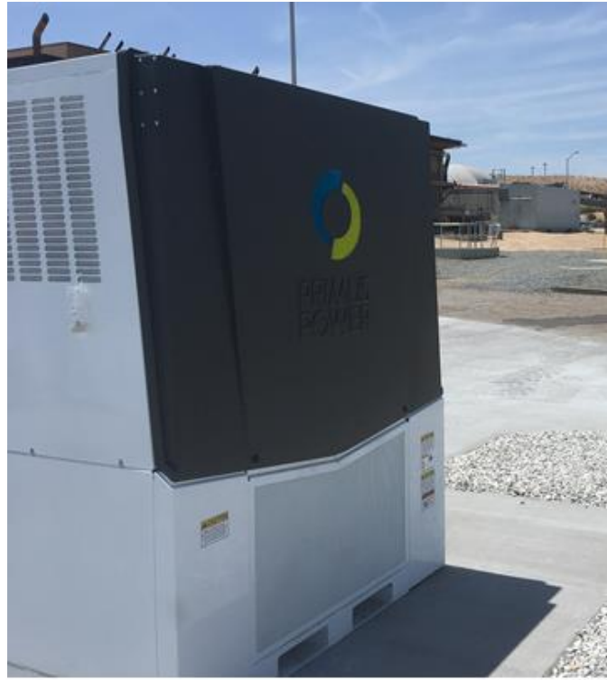
Primus Power EnergyPod2 flow battery installed at VVWRA.
