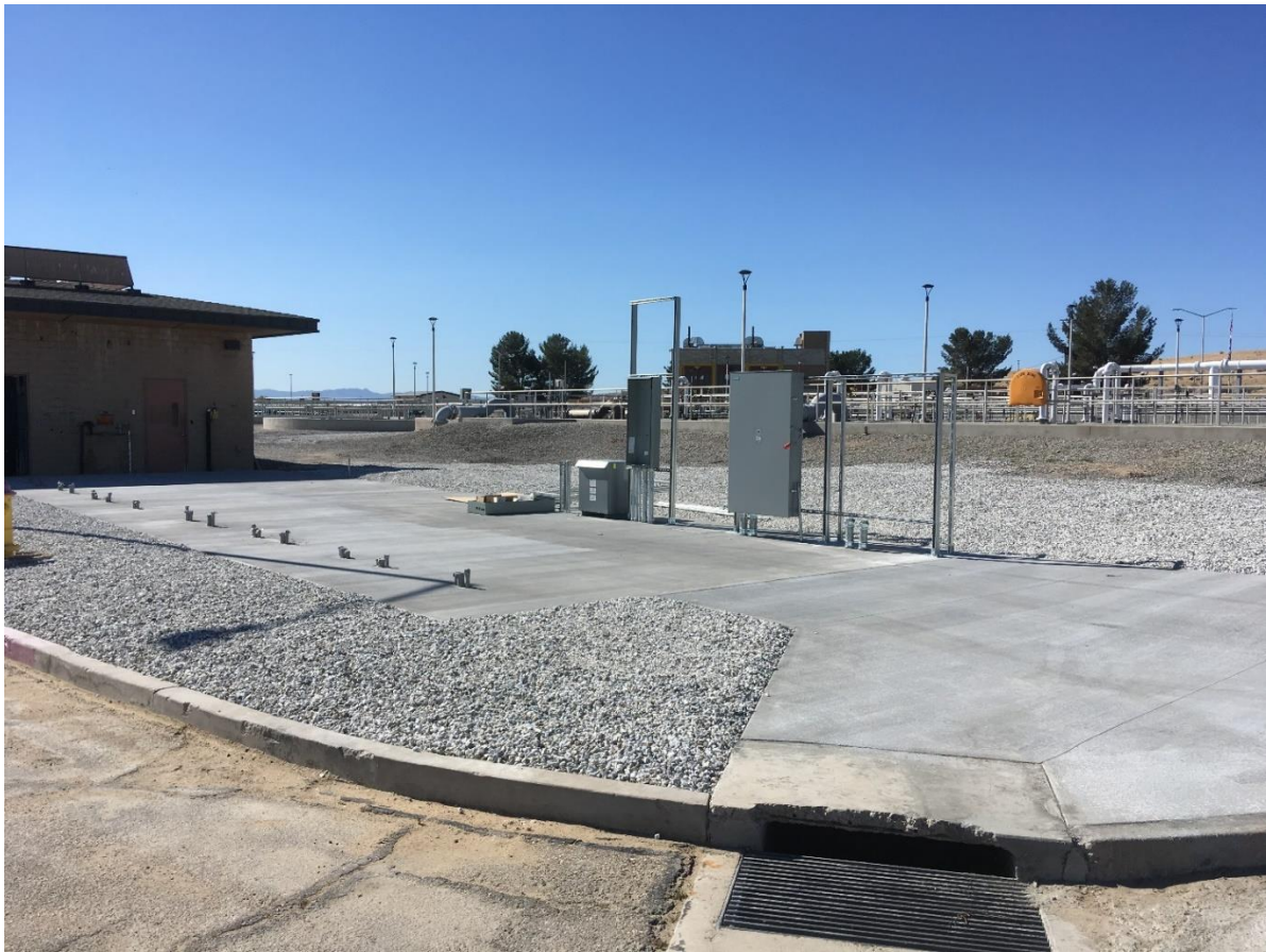
Figure 9: Prepared Flow Battery Foundation
