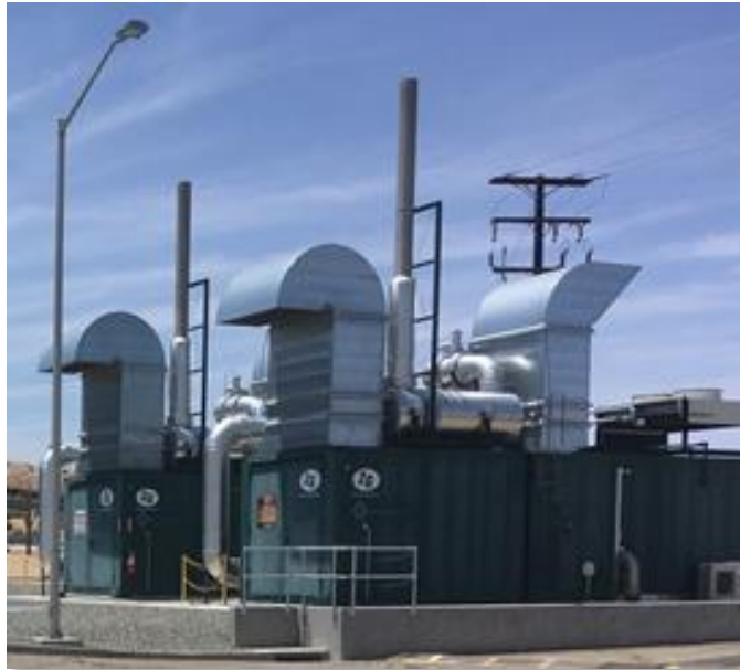
Two 800-kW renewable energy generators.
