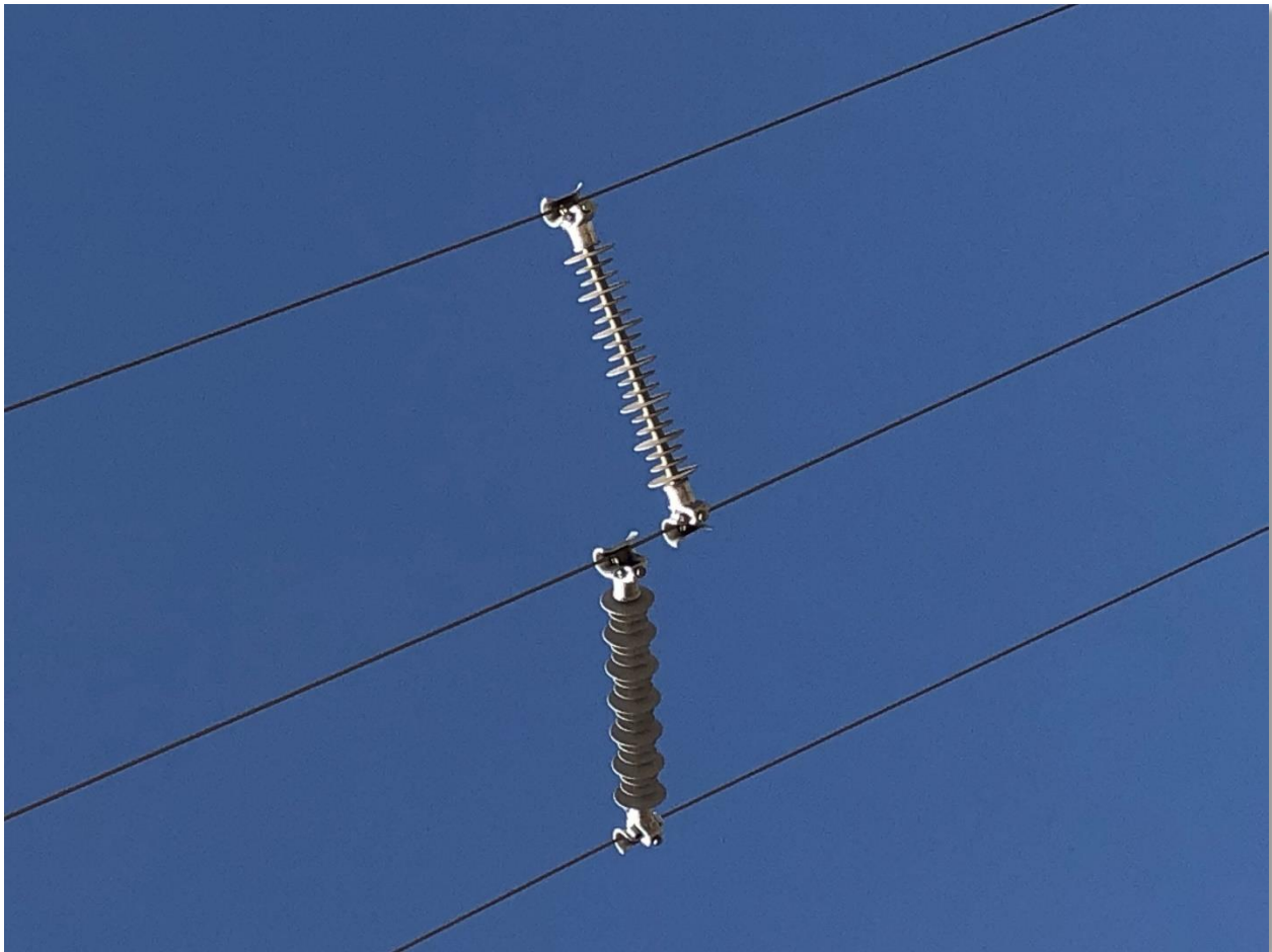
Figure 14: Line Spacers on Utility Wires
