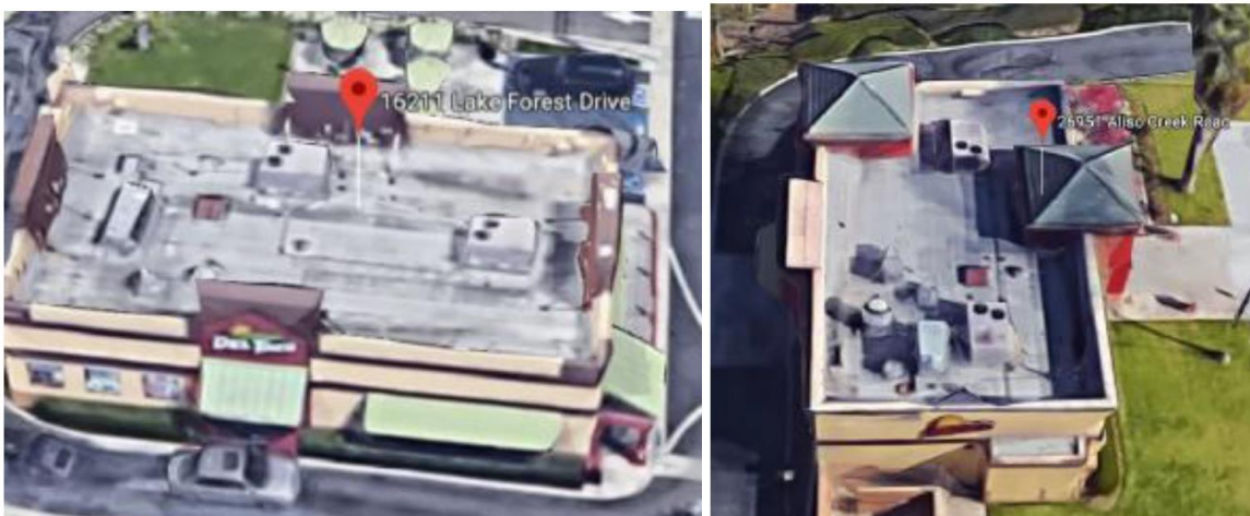
Figure 19: Rooftop Views Del Taco Treatment (left) and Control (right) Sites
