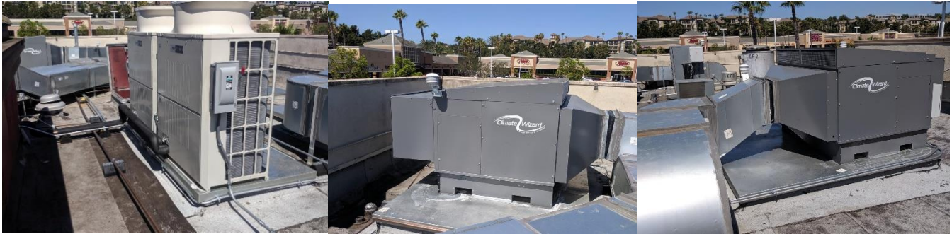
Figure 33: Variable Refrigerant Flow and Indirect Evaporative Cooling Units Installed on Roof of Del Taco
