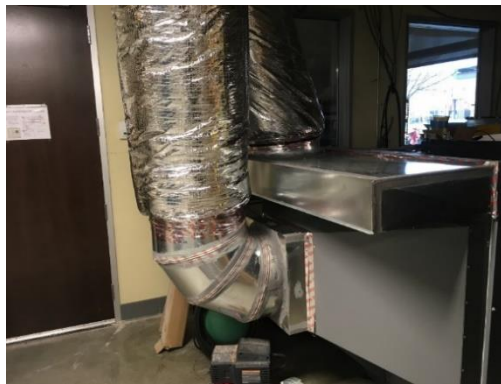
Figure 28: Completed Indirect Evaporative Cooling Supply and Exhaust Connections
