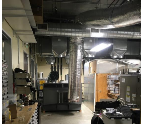
Figure 27: Indirect Evaporative Cooling Insulated Supply Flex Duct During Construction
