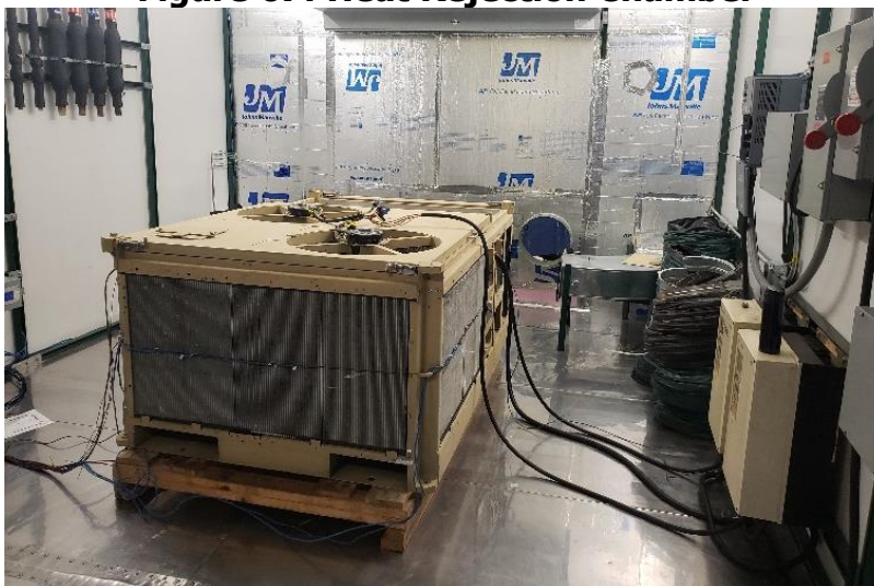
Figure 67: Heat Rejection Chamber
