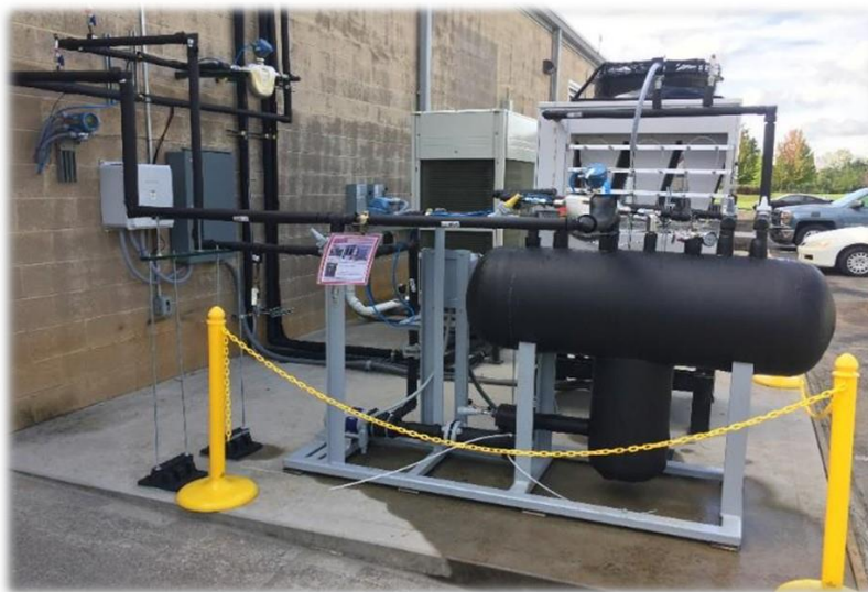
Figure 74: Outdoor System Fully Installed
