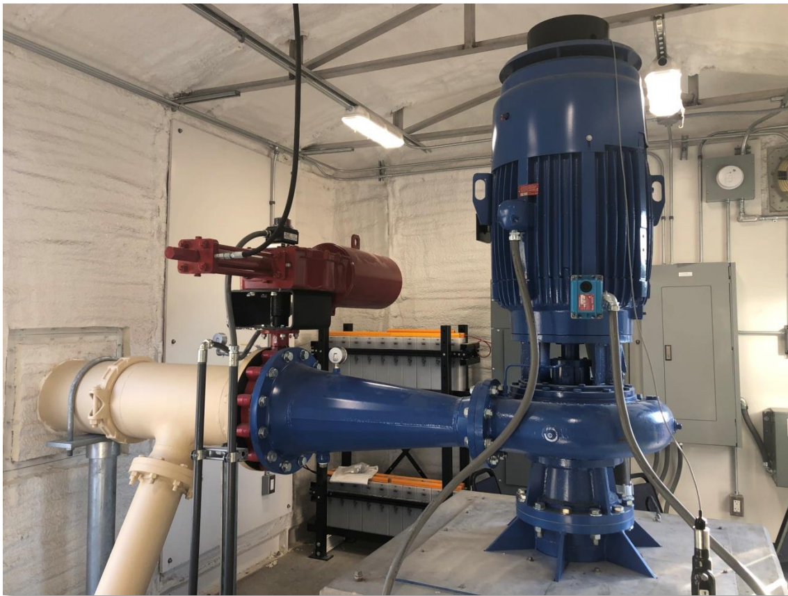
Figure 5: Cornell Pump-as Turbine-Generator in Vertical Configuration at B24
