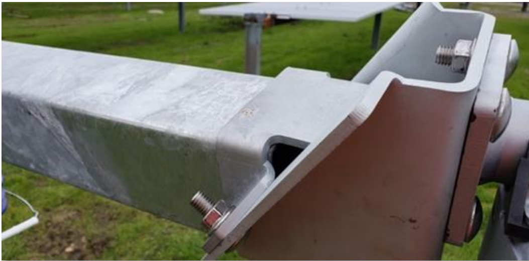
Figure 30: 1" Minimum Engagement Necessary to Retain the Torque Tube in High Wind Conditions
