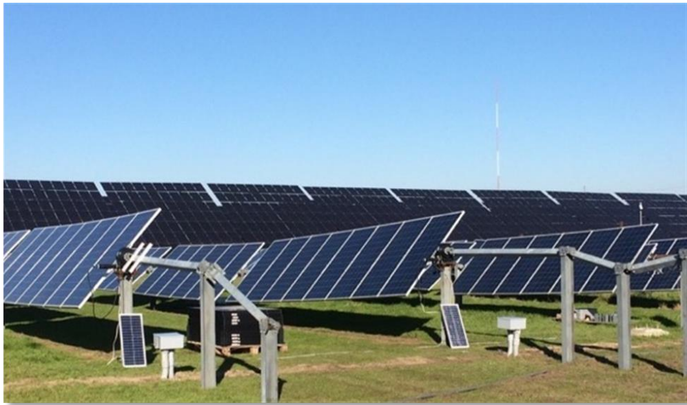
Figure 1: Nevados Test Site Shows Exposed Module Mounting Tube and Allowable Angles
