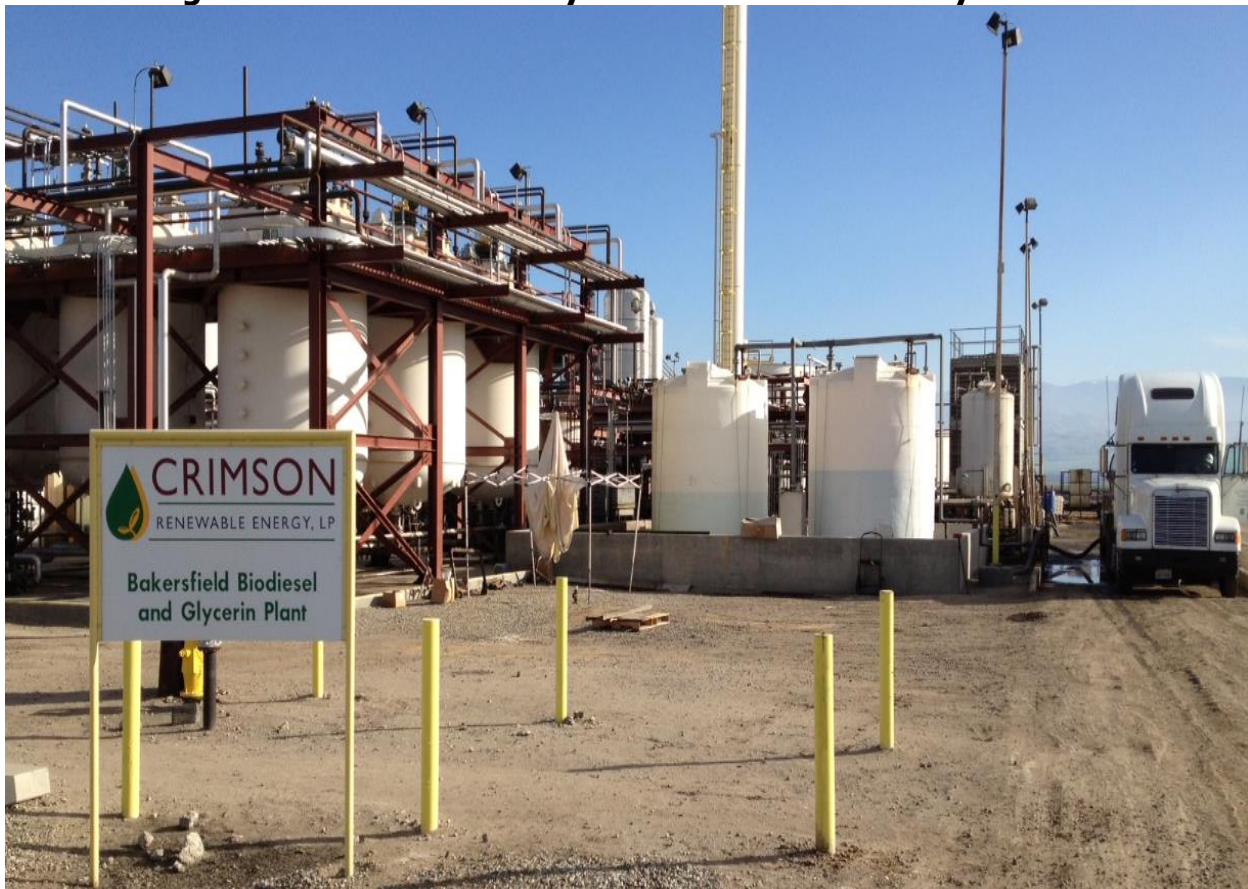
Figure 1: Biodiesel and Glycerin Production Facility in 2013
