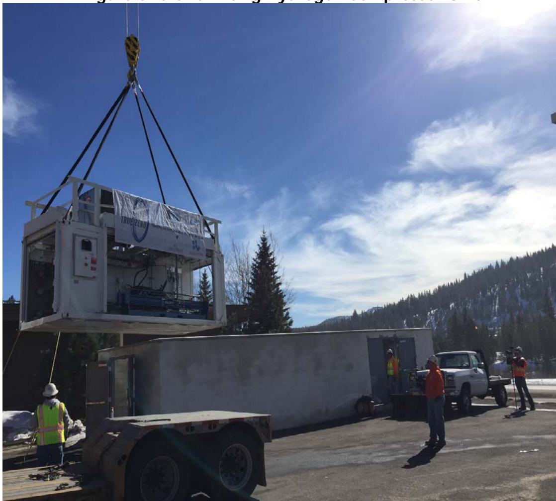
Figure 6: Crane Lifting Hydrogen Compressor Unit
