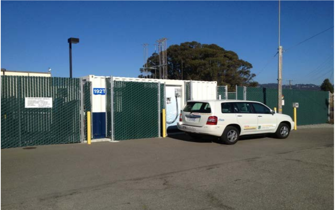
Figure 4: 700-Bar Hydrogen Fueling Dispenser at the UC Berkeley Richmond Field Station
