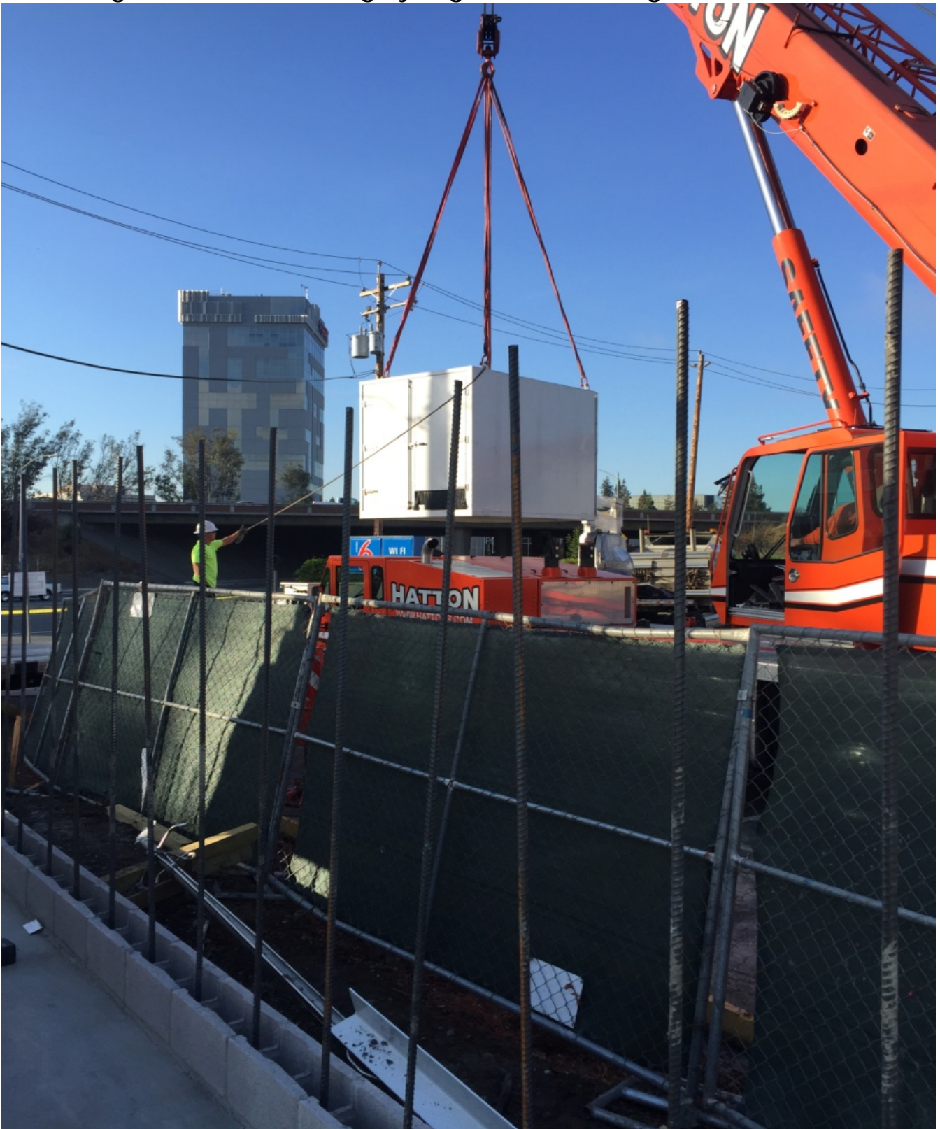
Figure 5: Crane Lowering Hydrogen Ground Storage Unit into Place
