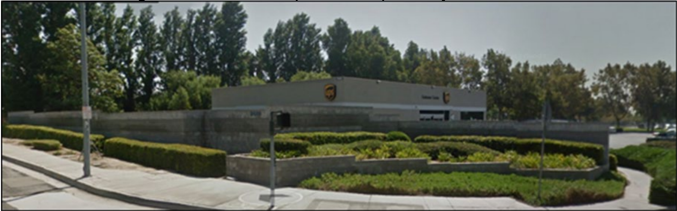
Figure 9: UPS Ontario, California, Facility
