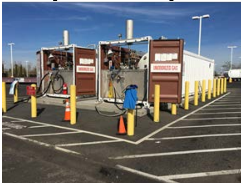
Figure 6: Installed Fueling Units
