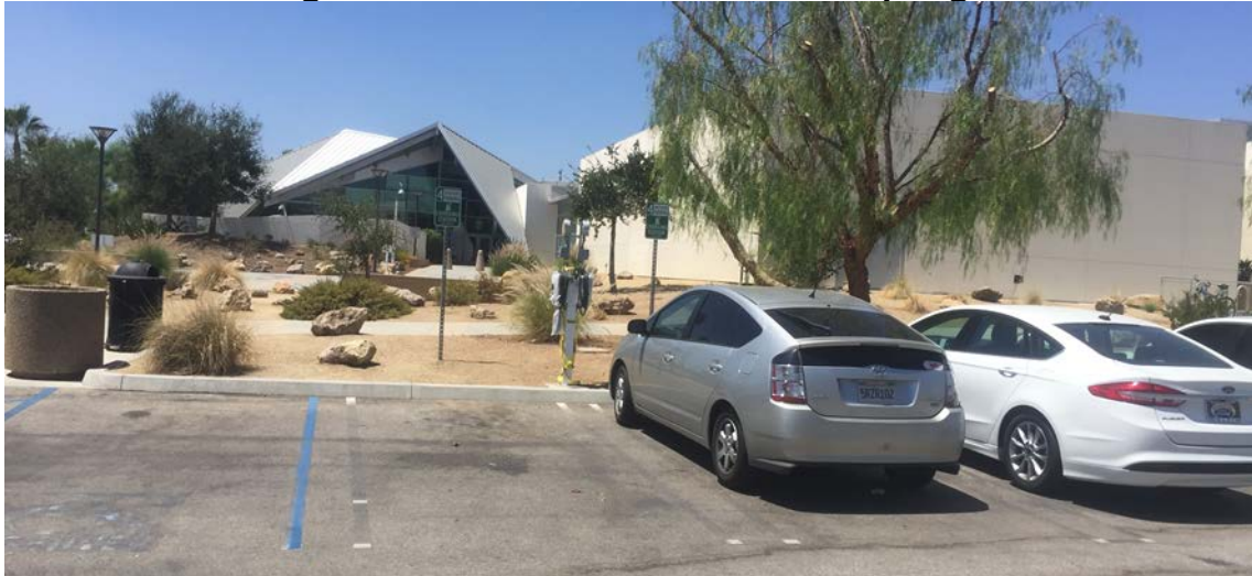
Figure 15: Installation at LAPD: Topanga
