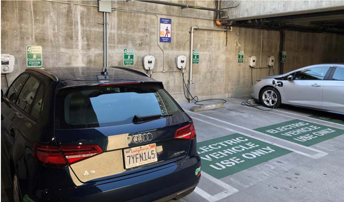
Figure 2: Installation at LADOT: Aiso
