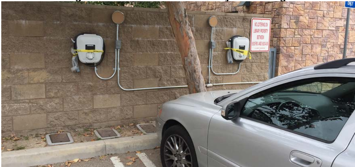
Figure 23: Installation at Library: Northridge
