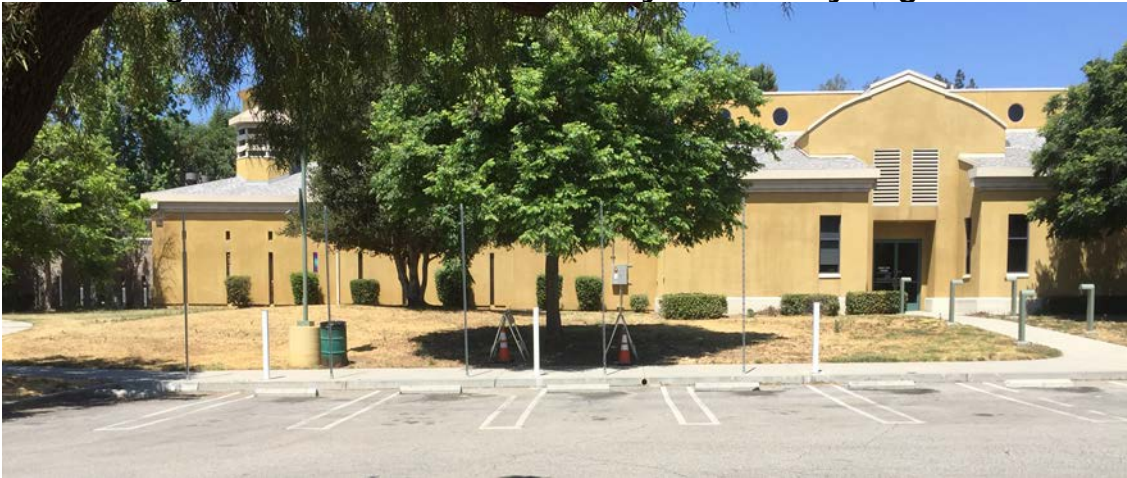
Figure 22: Installation at Library: Mid Valley Regional
