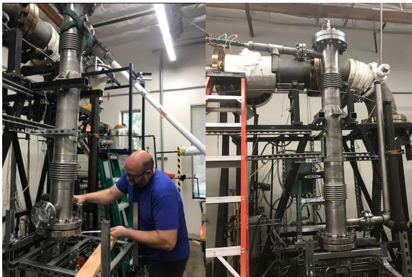
Figure 35: Fuel Production Reactor Installation (Left) and the Installed Unit (Right)
