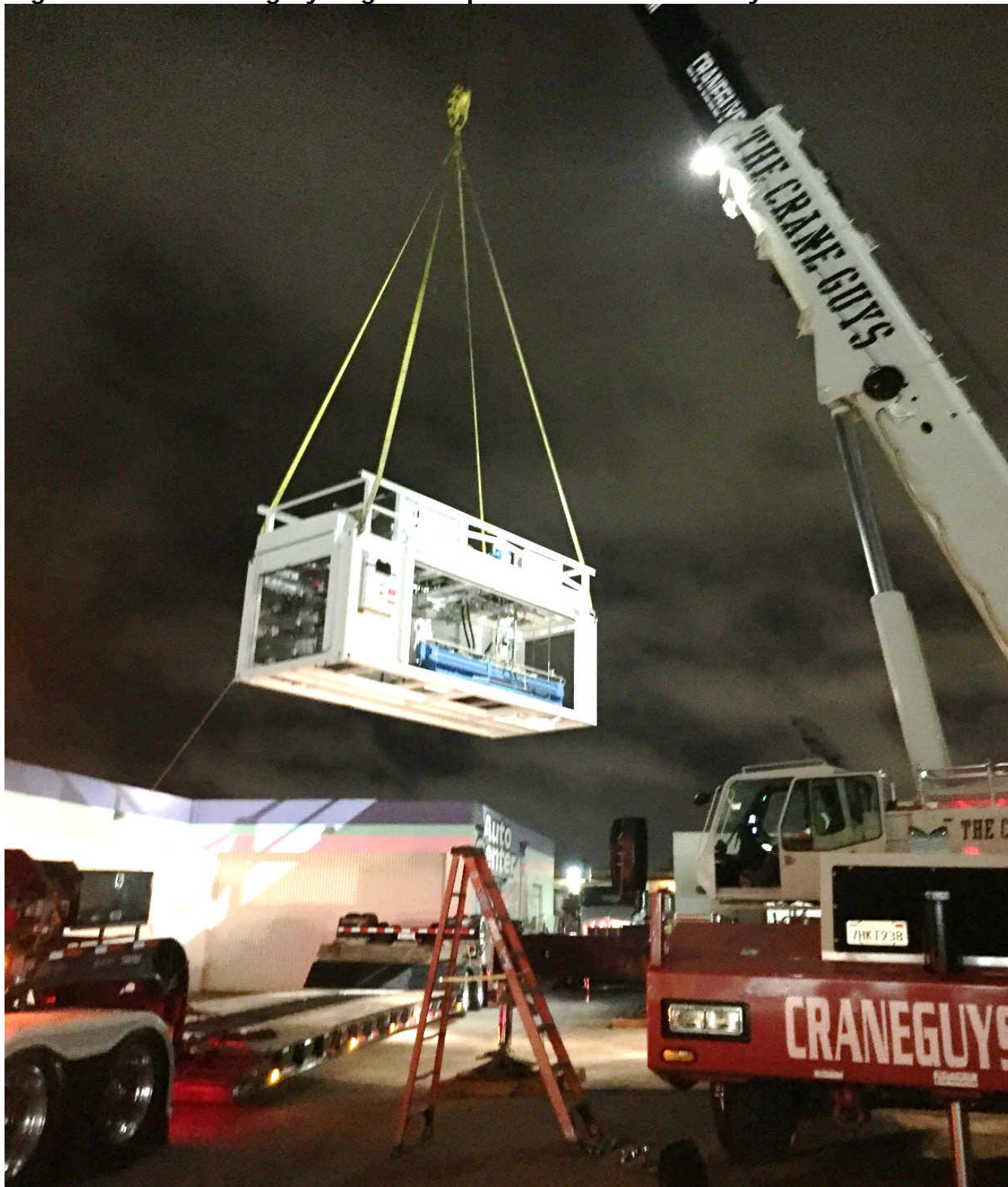
Figure 2: Crane Lifting Hydrogen Compressor Unit off Delivery Truck in Costa Mesa
