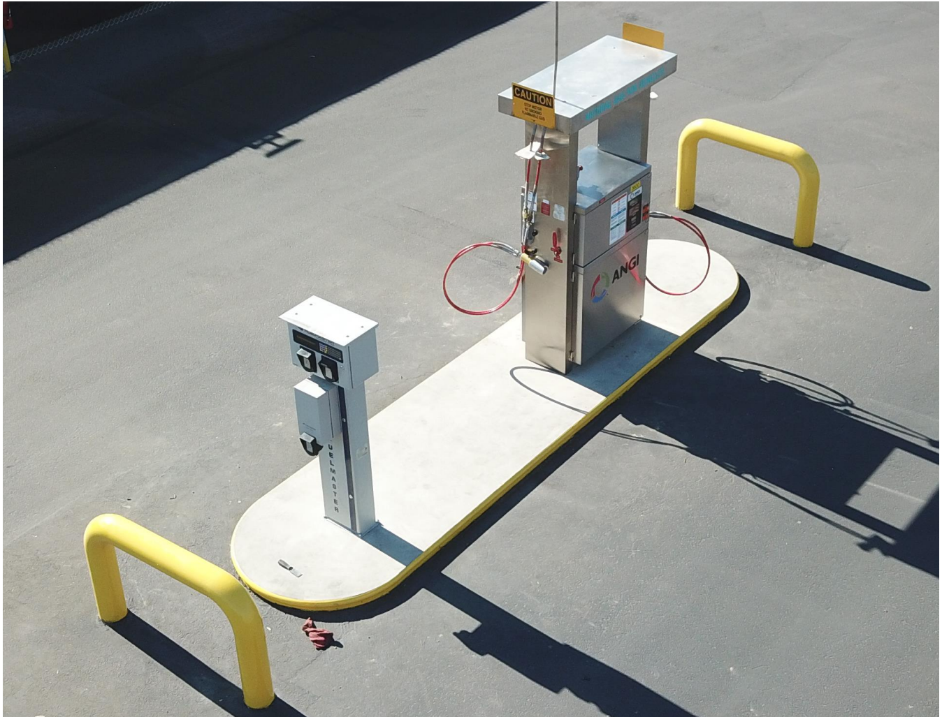
Figure 3: New Dual Hose Fast-Fill Dispenser
