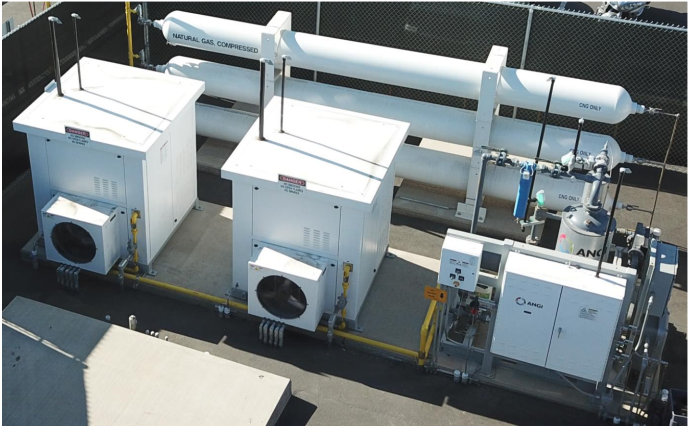
Figure 1: HBUHSD CNG Refueling Station—Two 50-HP Compressors
