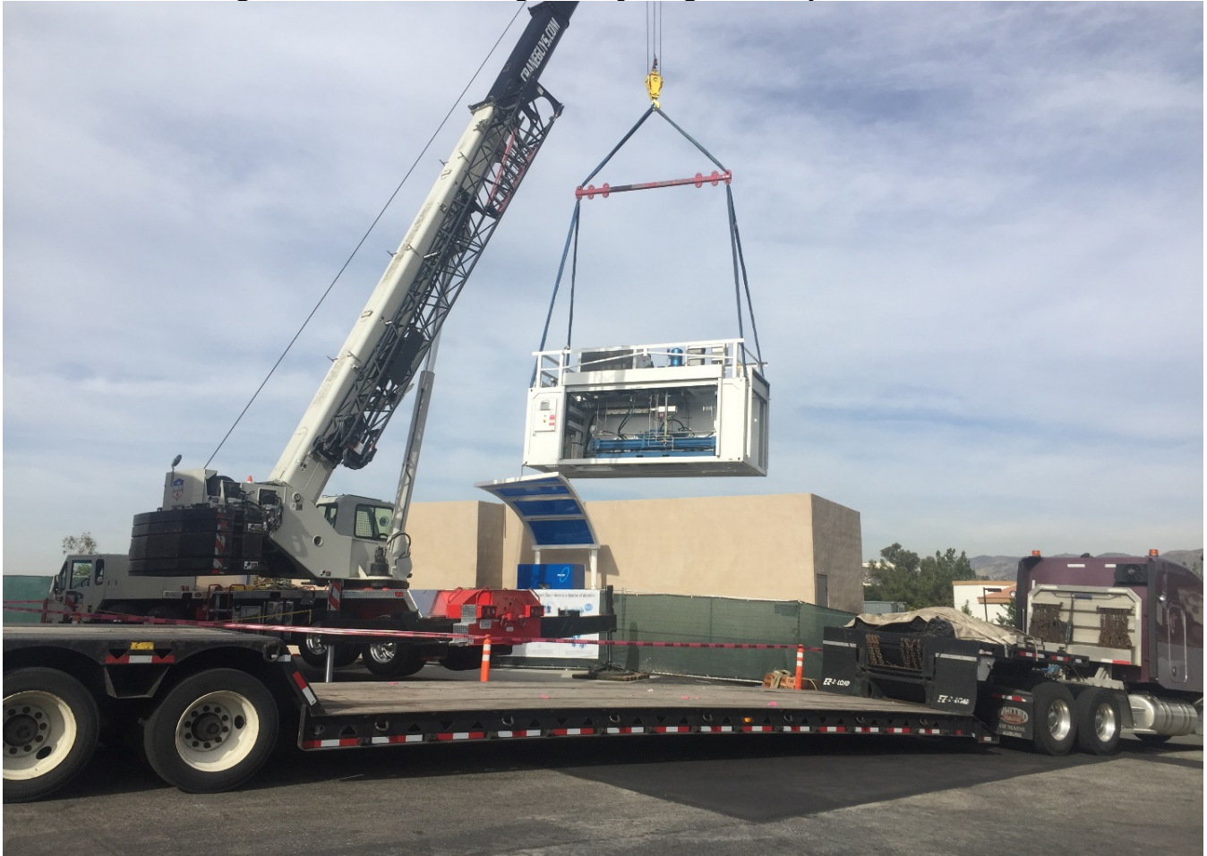
Figure 6: Crane Lifting the Hydrogen Compression Unit
