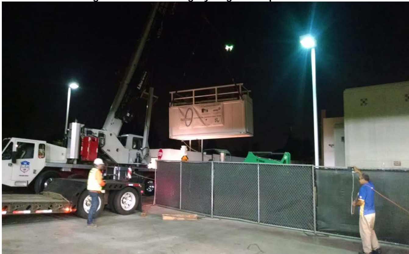
Figure 6: Crane Lifting Hydrogen Compressor Unit
