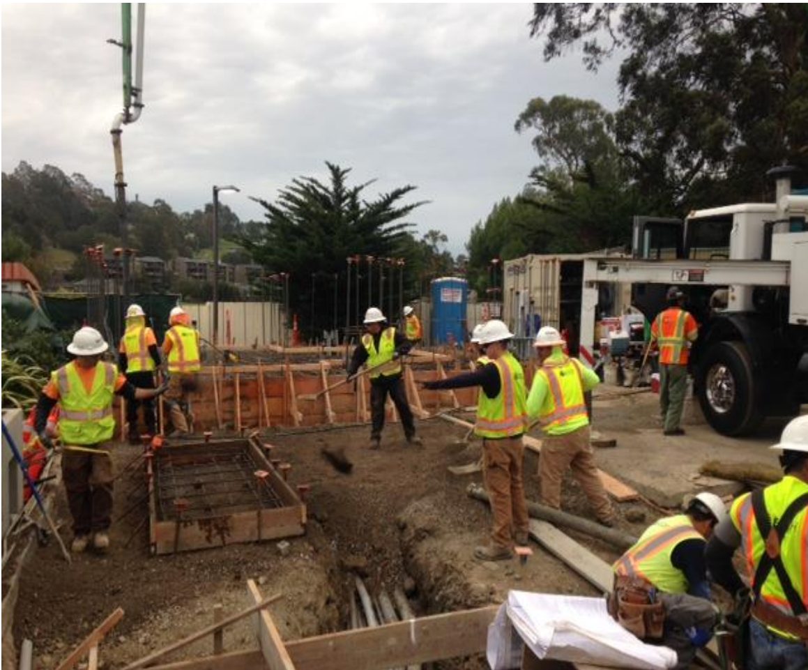
Figure 5: Concrete Formwork in Progress
