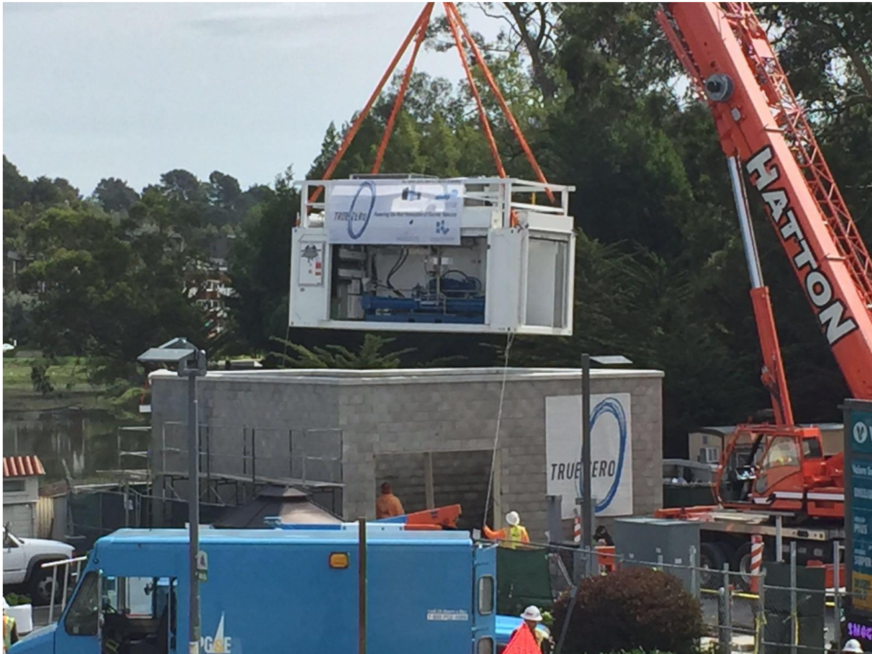
Figure 6: Crane Lifting Hydrogen Compression Unit
