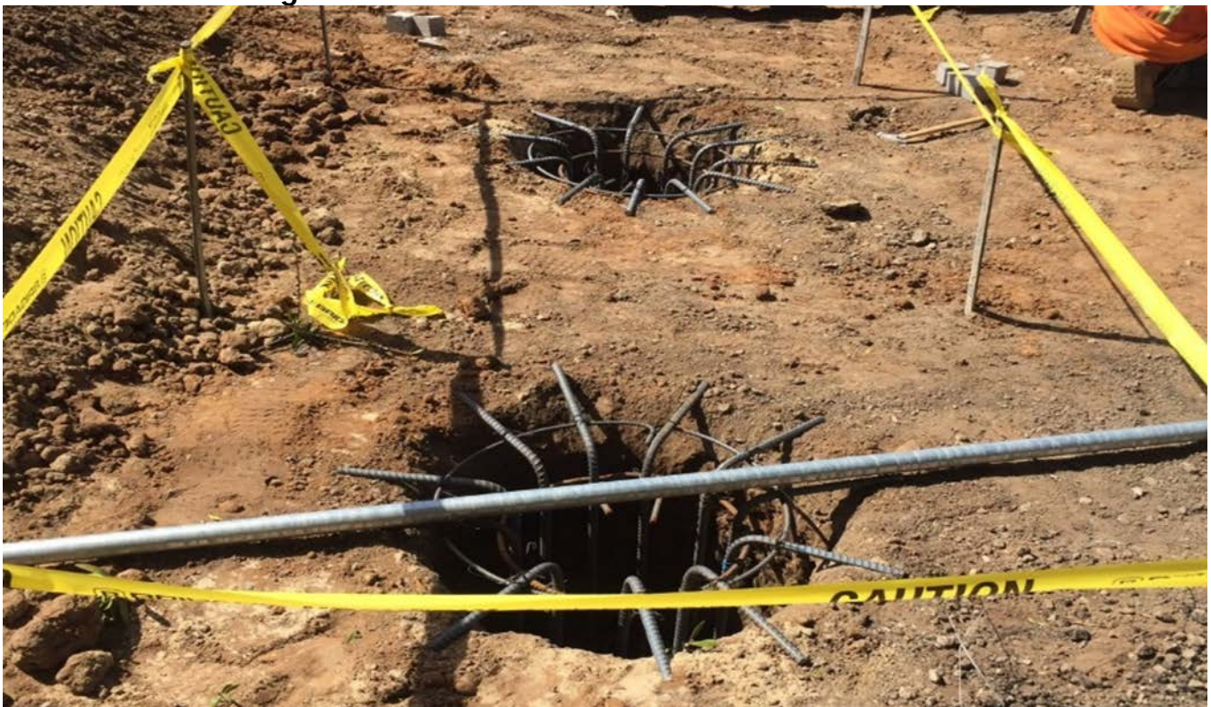
Figure 4: Rebar Installation for Pier Foundations
