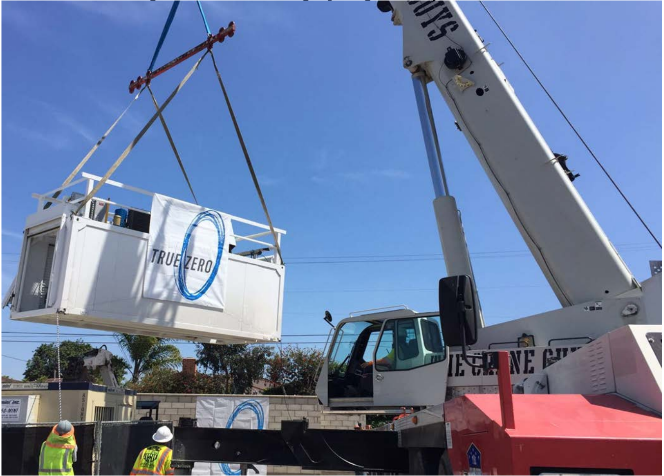
Figure 5: Crane Lifting Hydrogen Compressor Unit
