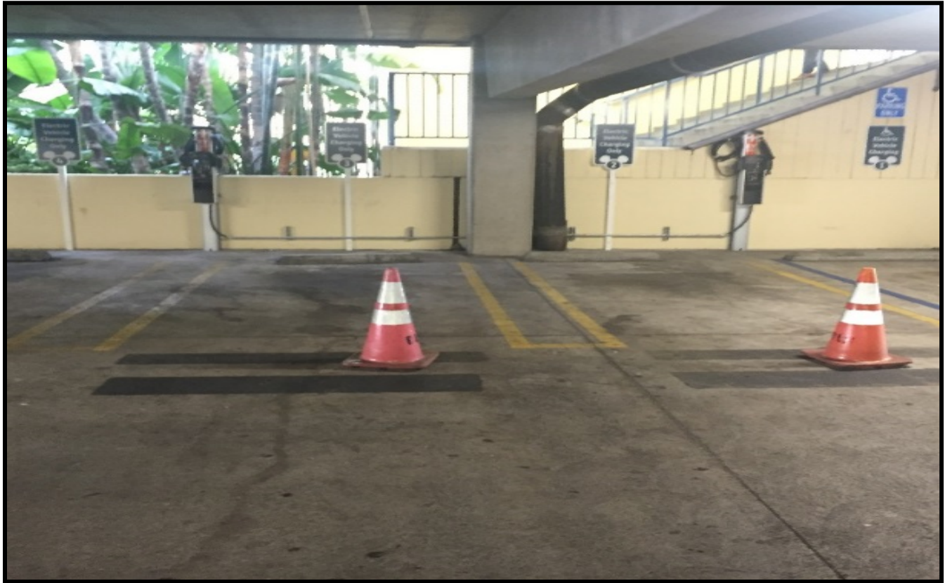
Figure 11: Installed EV charging stations at Paradise Pier Hotel parking garage
