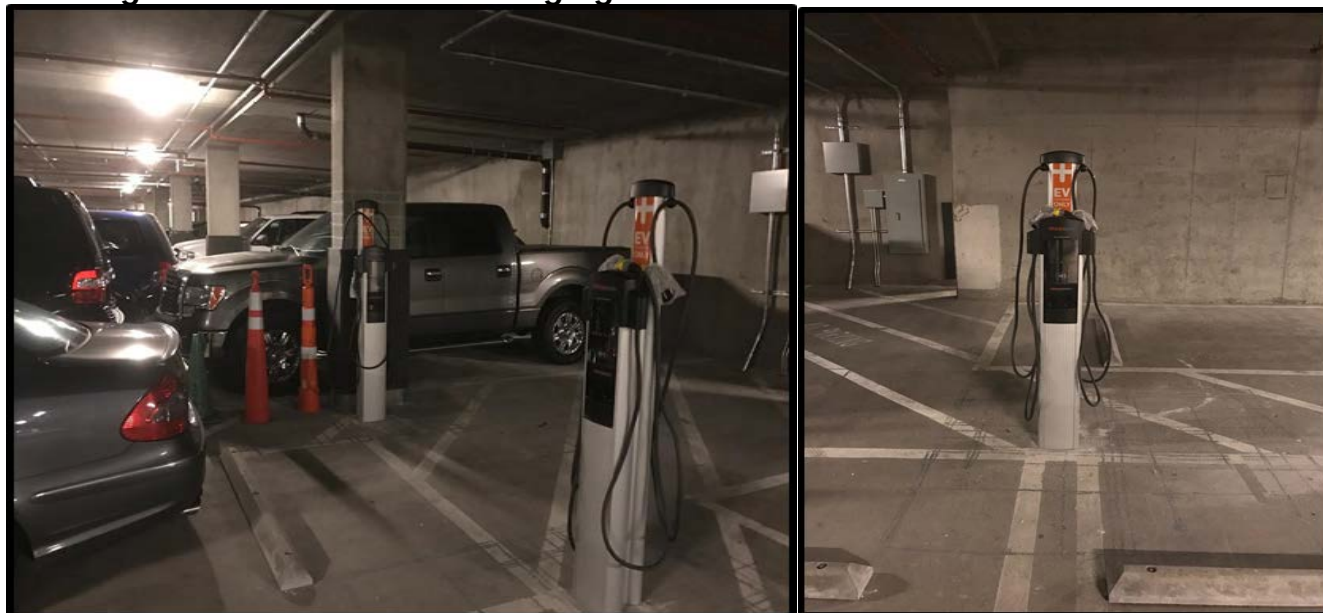
Figure 18: Installed EV Charging Stations at the Grand Californian Hotel
