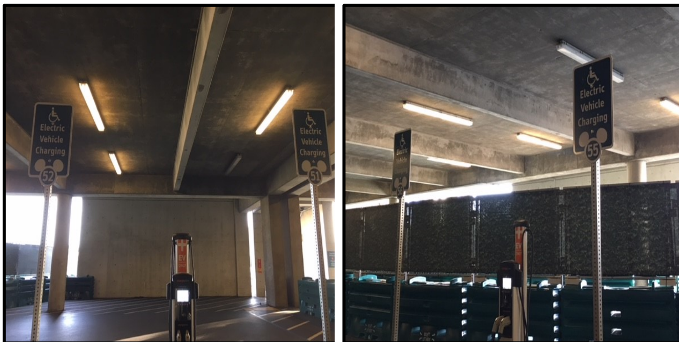
Figure 9: Installed ADA Compliant EV charging stations on Level 1 Mickey & Friends Parking Structure
