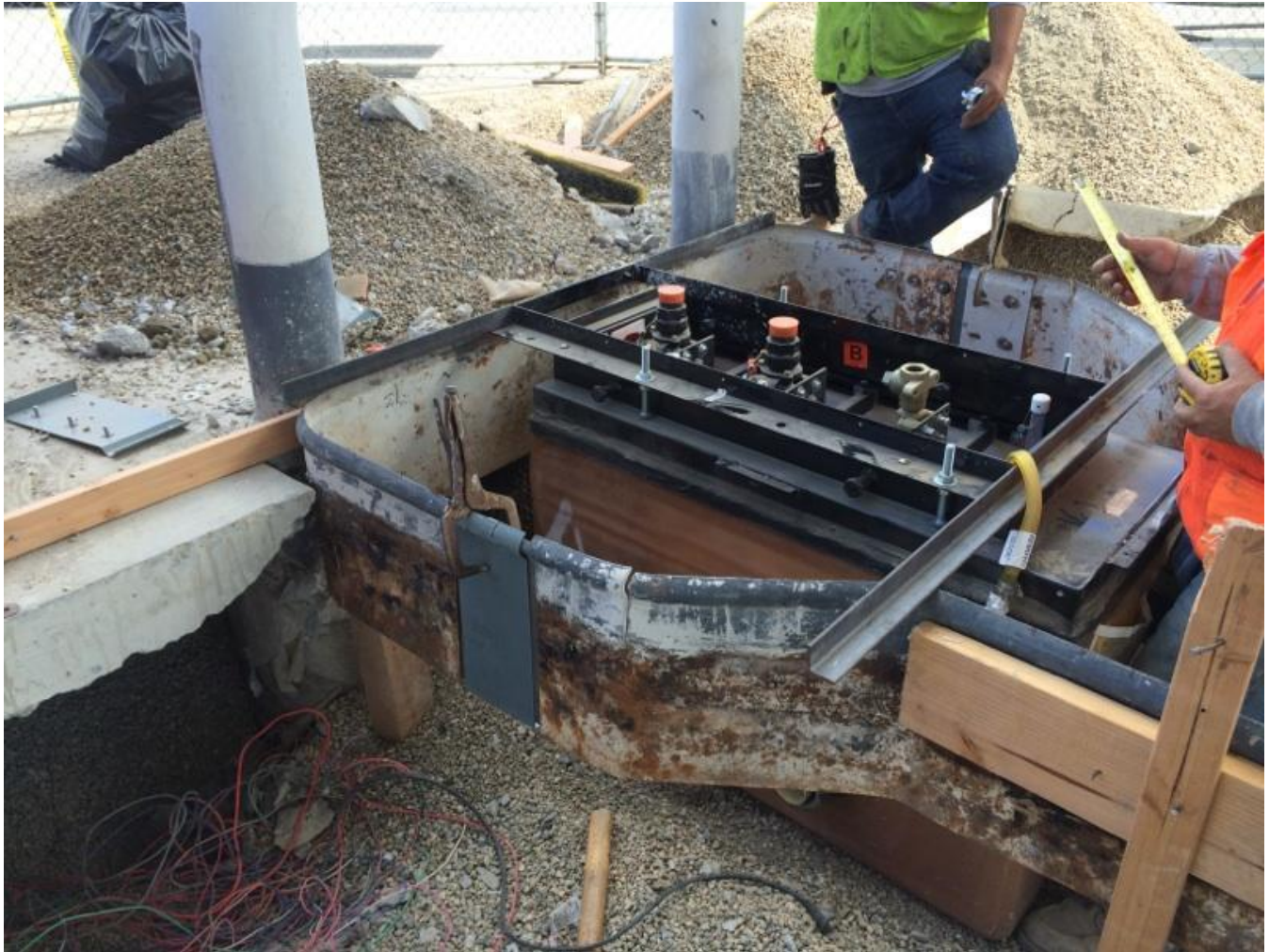
Figure 8: Lakewood - Under Dispenser Containment and Island Form
