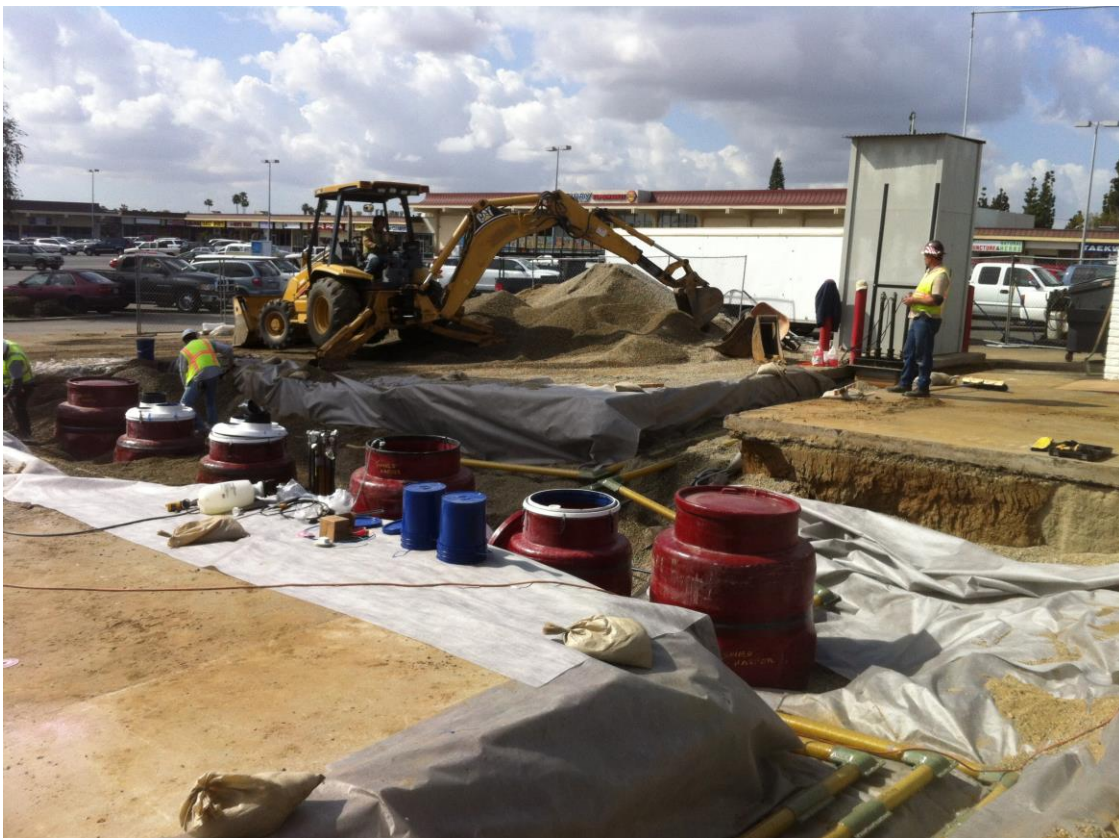
Figure 7: La Mirada – Installation of Sumps and Piping
