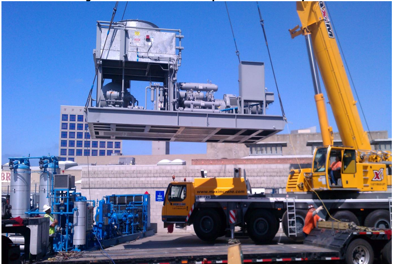
Figure 1: Installation of Compressor and Gas Dryer
