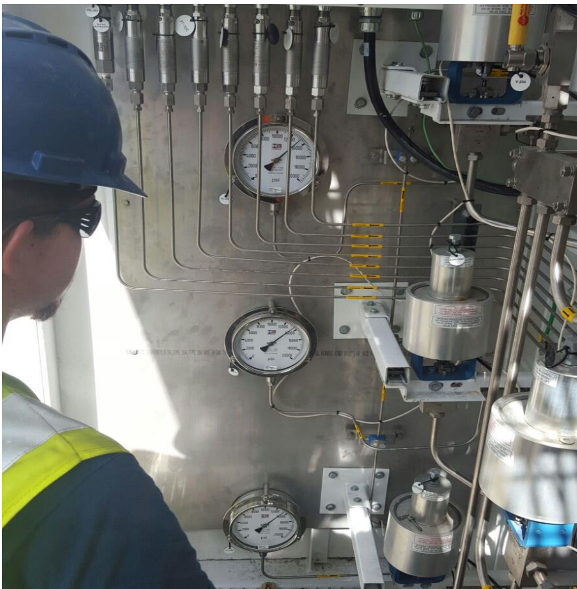
Figure 7: Technician Conducting First Pressure Test during Commissioning
