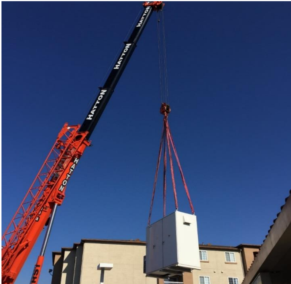
Figure 6: Crane Lifting Electrical Cabinet
