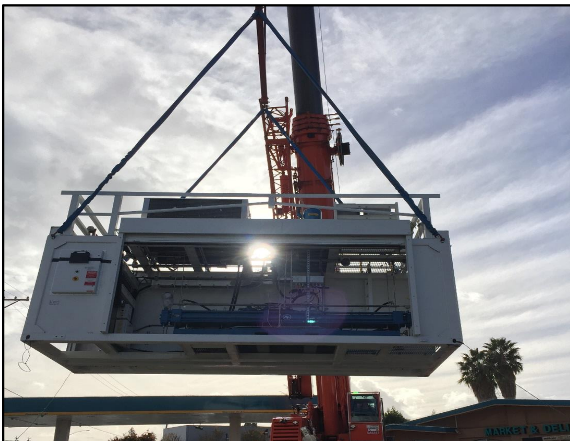
Figure 4: Crane Lifting Hydrogen Compressor Unit
