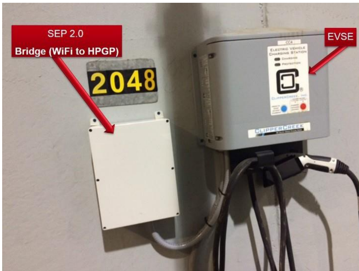
Figure 123: Communication Box Connected to EVSE
