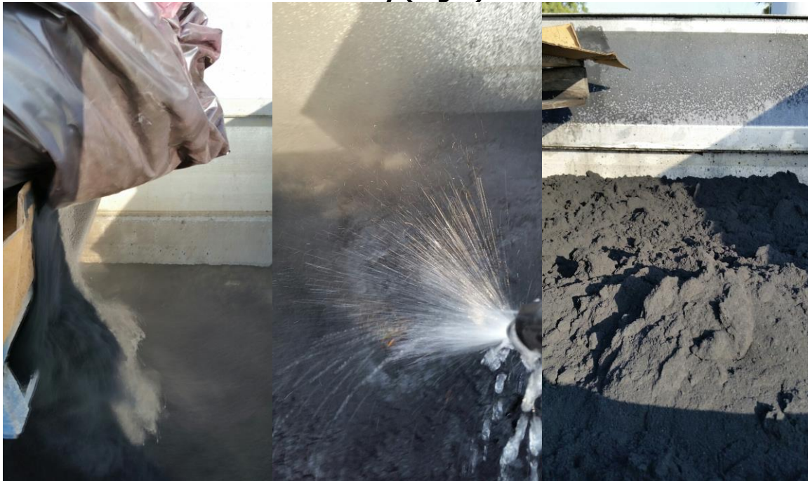
Figure 22: Pouring Biochar Into Hopper (Left), Dust Control (Middle), Resulting Slurry (Right)
