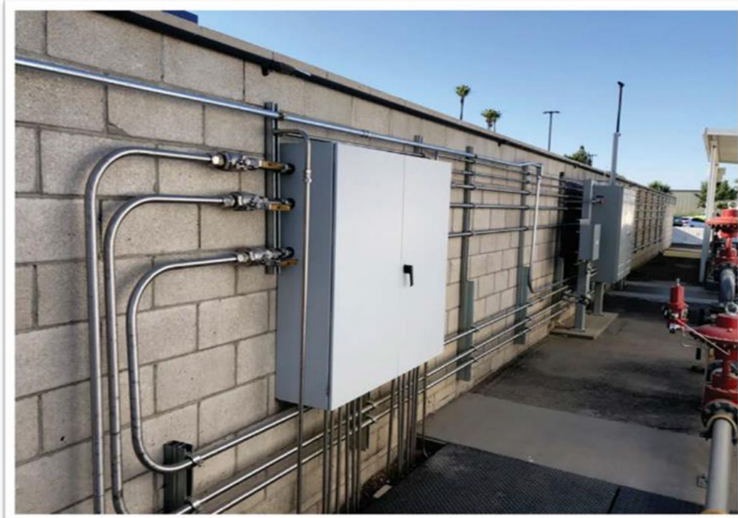
Figure 9: CNG Piping and Electrical Conduit
