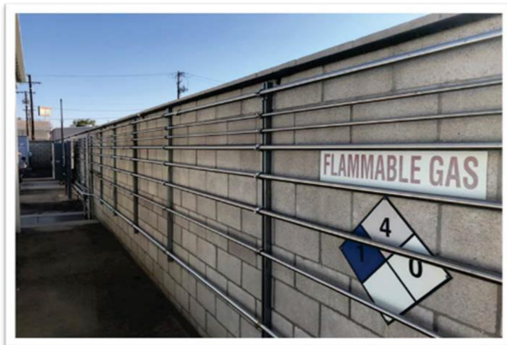
Figure 10: CNG Piping and Electrical Conduit
