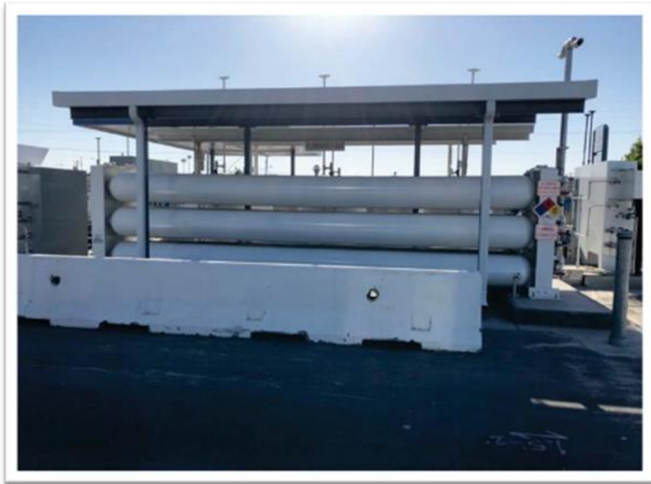
Figure 11: CNG Storage Tanks with Canopy
