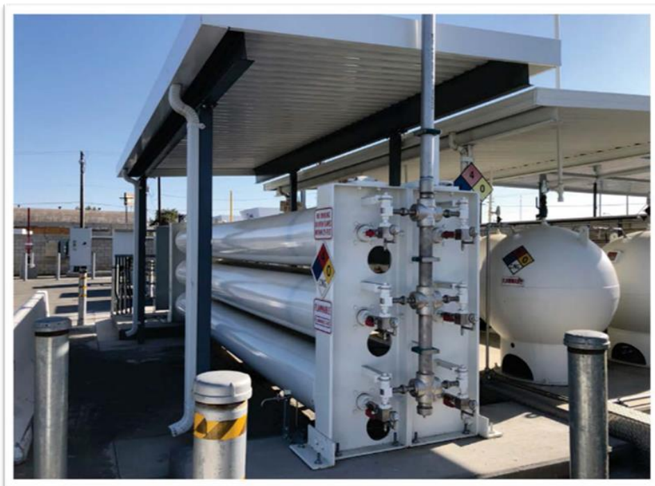
Figure 12: CNG Storage Tanks with Canopy
