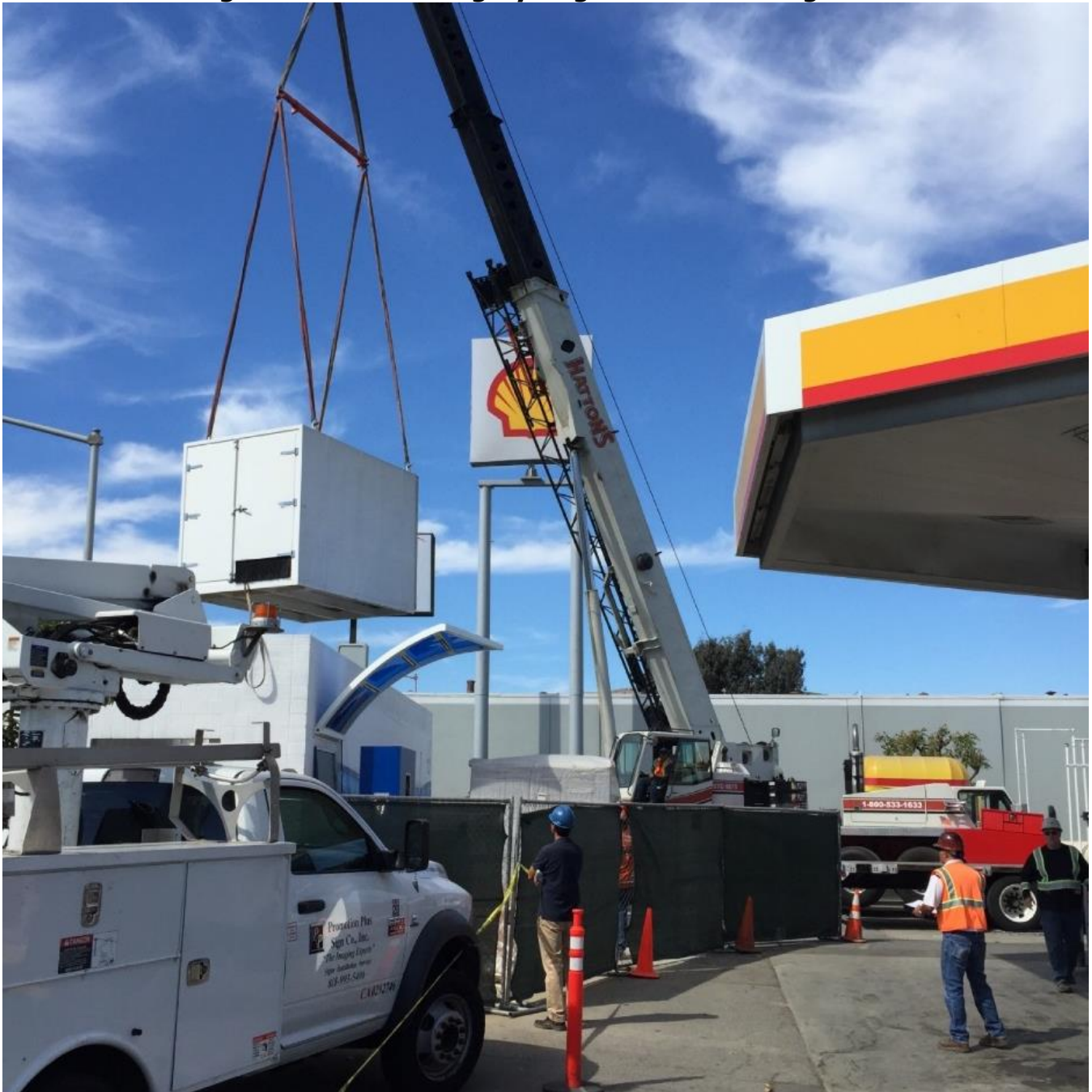
Figure 6: Crane Lifting Hydrogen Ground Storage Unit
