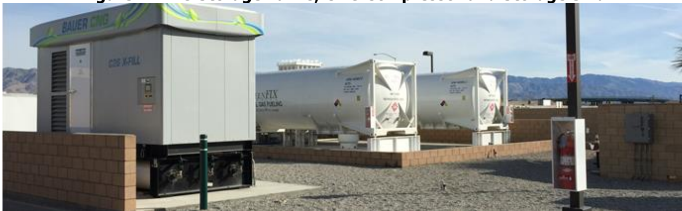
Figure 4: LNG Storage Tanks, CNG Compressor and Storage Skid
