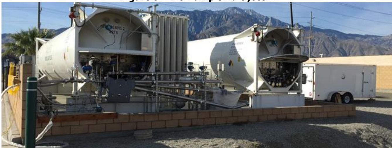
Figure 5: LNG Pump Skid System
