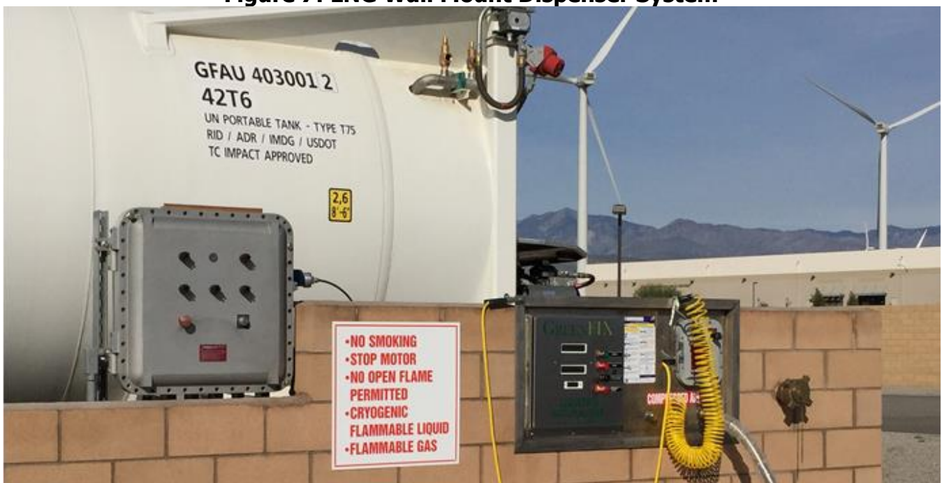
Figure 7: LNG Wall Mount Dispenser System
