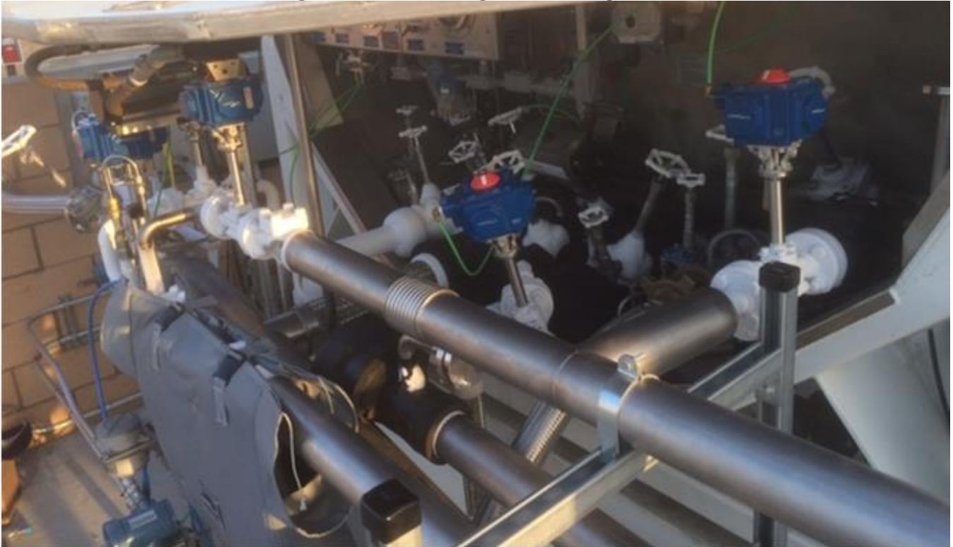
Figure 6: Plumbing for LNG System
