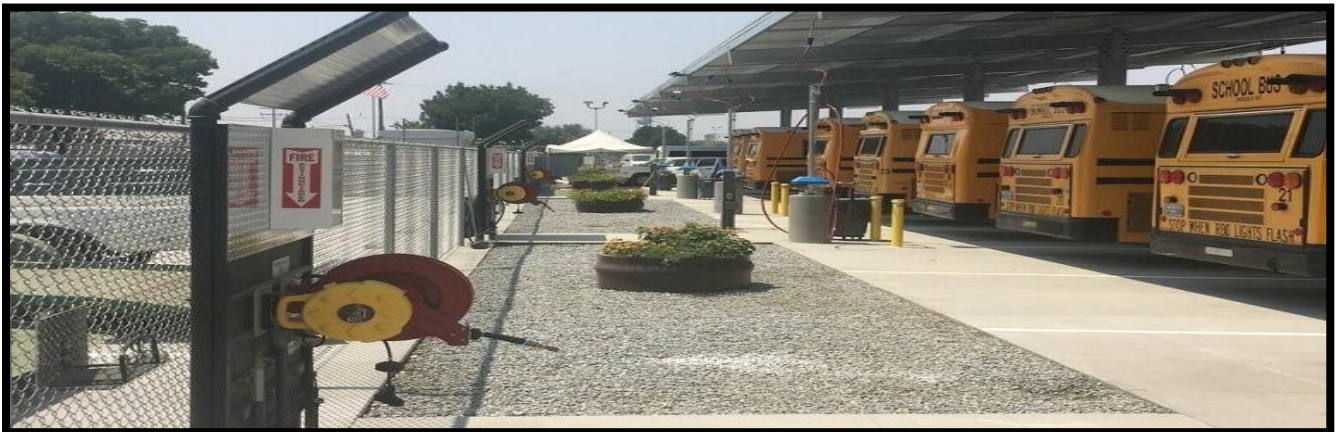
Figure 3: Upgraded Shade and Electrical
