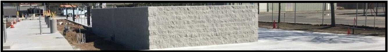
Figure 5: Concrete Wall Surrounding Equipment
