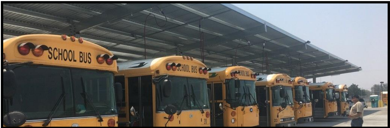
Figure 8: Completed Overhang Project
