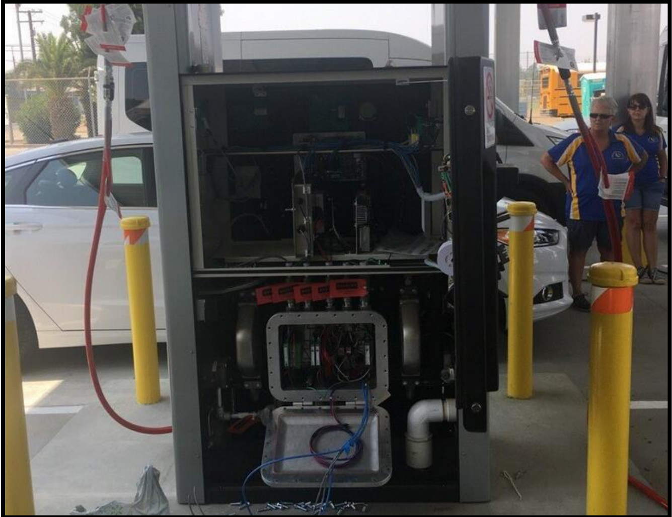
Figure B-7: Krauss Fast Fill Dispenser
