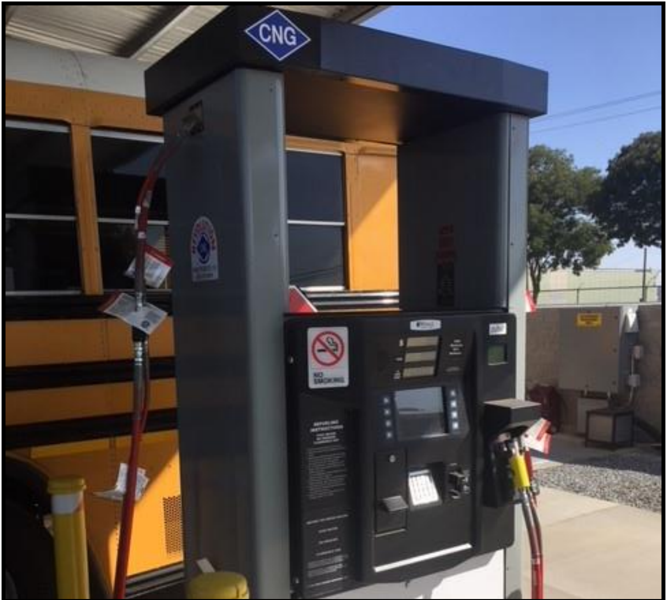
Figure B-6: Krauss Fast Fill Dispenser
