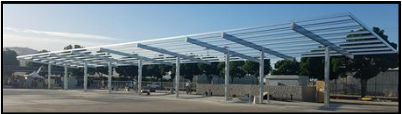
Figure 1: Construction of Fueling Stations
