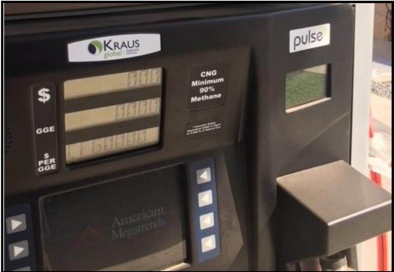
Figure B-9: Krauss Fast Fill Dispenser
