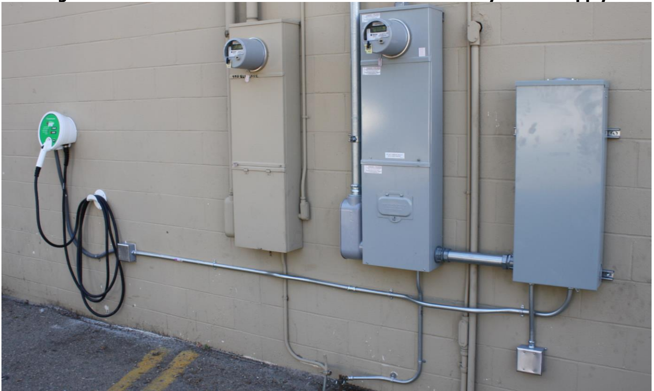
Figure 2: Low Cost Installation Wall Mounted with Nearby Power Supply
