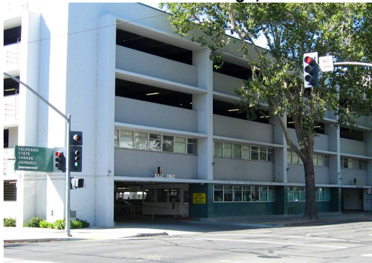
Figure 1: Sacramento State Garage, 1416 Tenth Street
