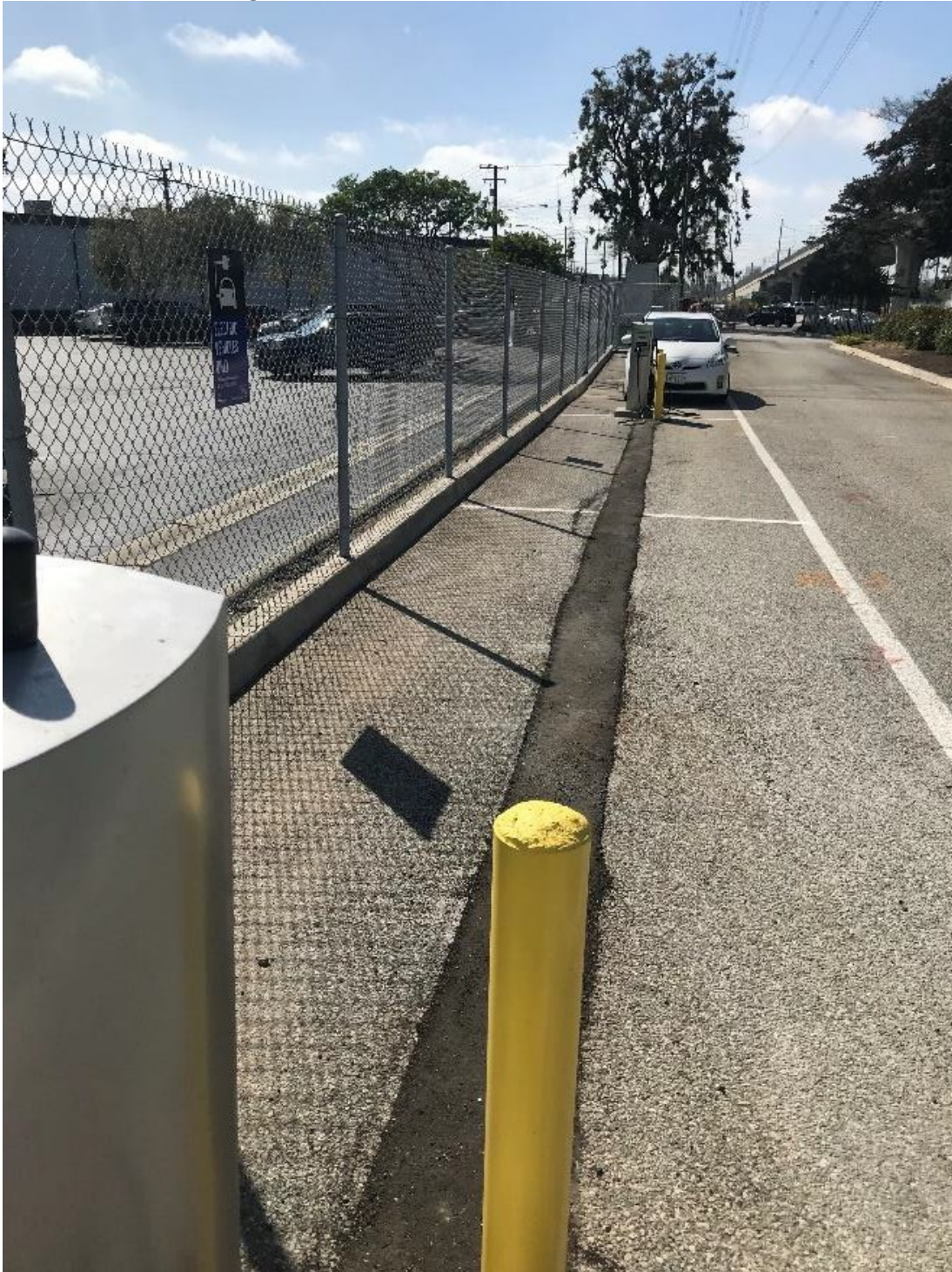
Figure 5: Redondo Beach Installation
