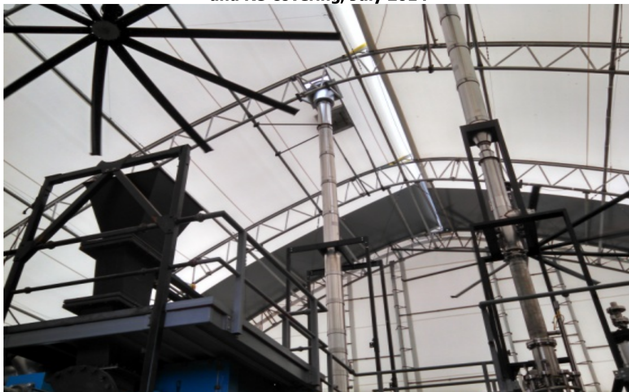
Figure 4: Installation of Custom Exhaust Flues After Roof Structure Modifications and Re-covering, July 2014
