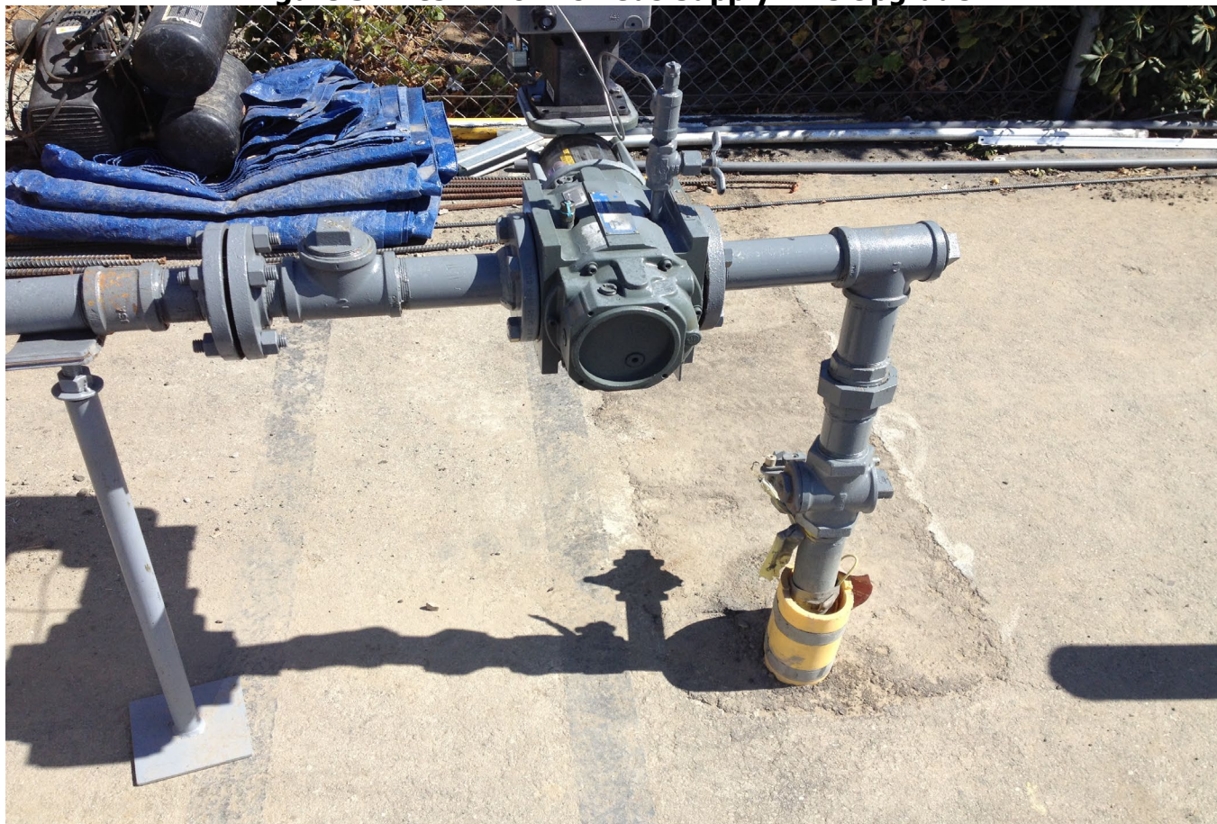
Figure 5: After Two Inch Gas Supply Line Upgrade
