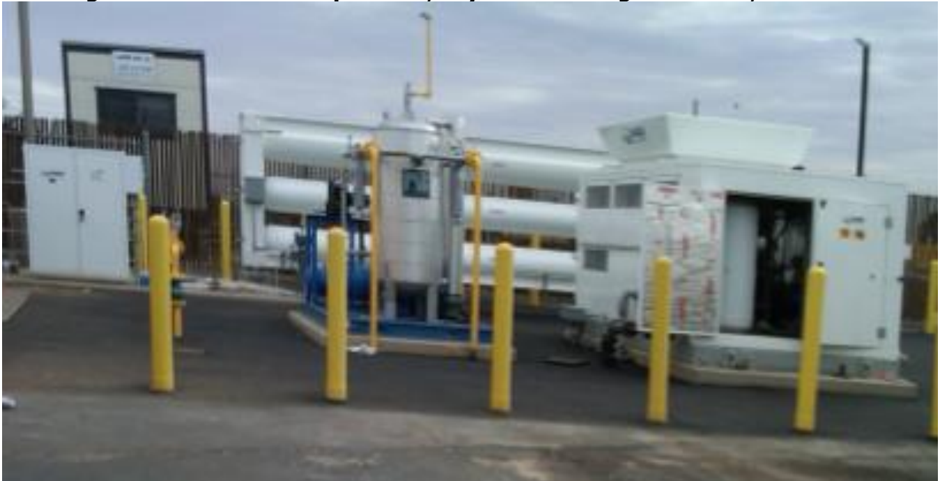
Figure 1: SoCalGas Compression, Dryer and Storage Facilities, Lancaster
