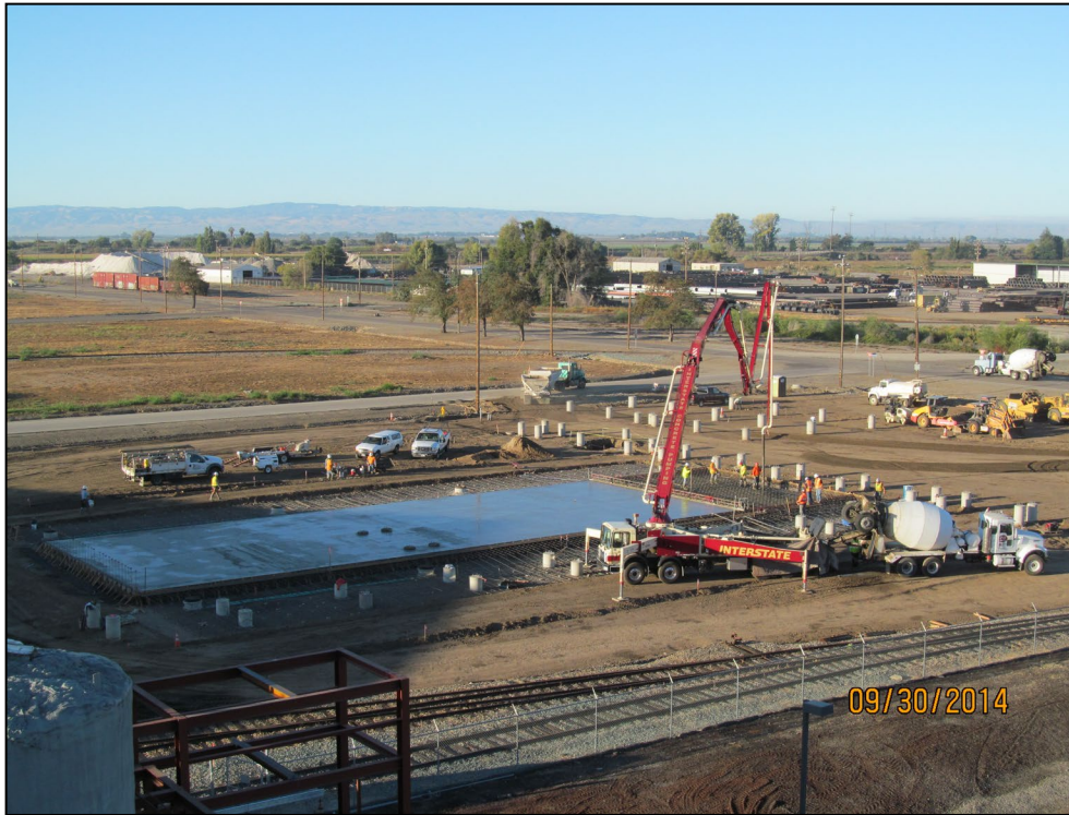
Figure 15: Concrete Finishing
