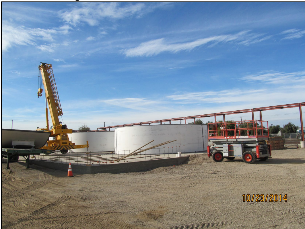
Figure 18: First Level of Tank Erection
