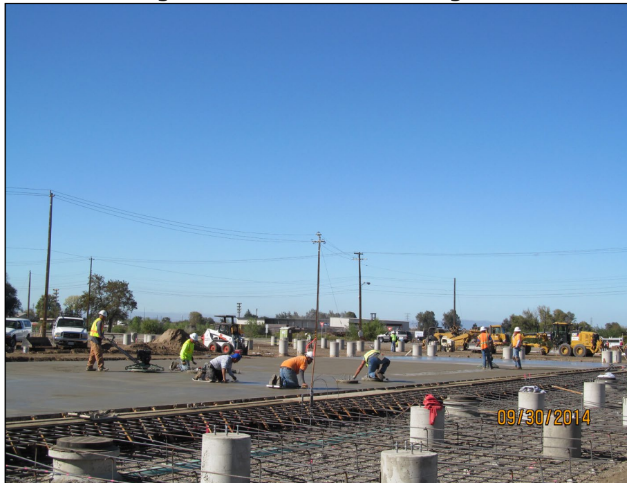
Figure 15: Concrete Finishing
