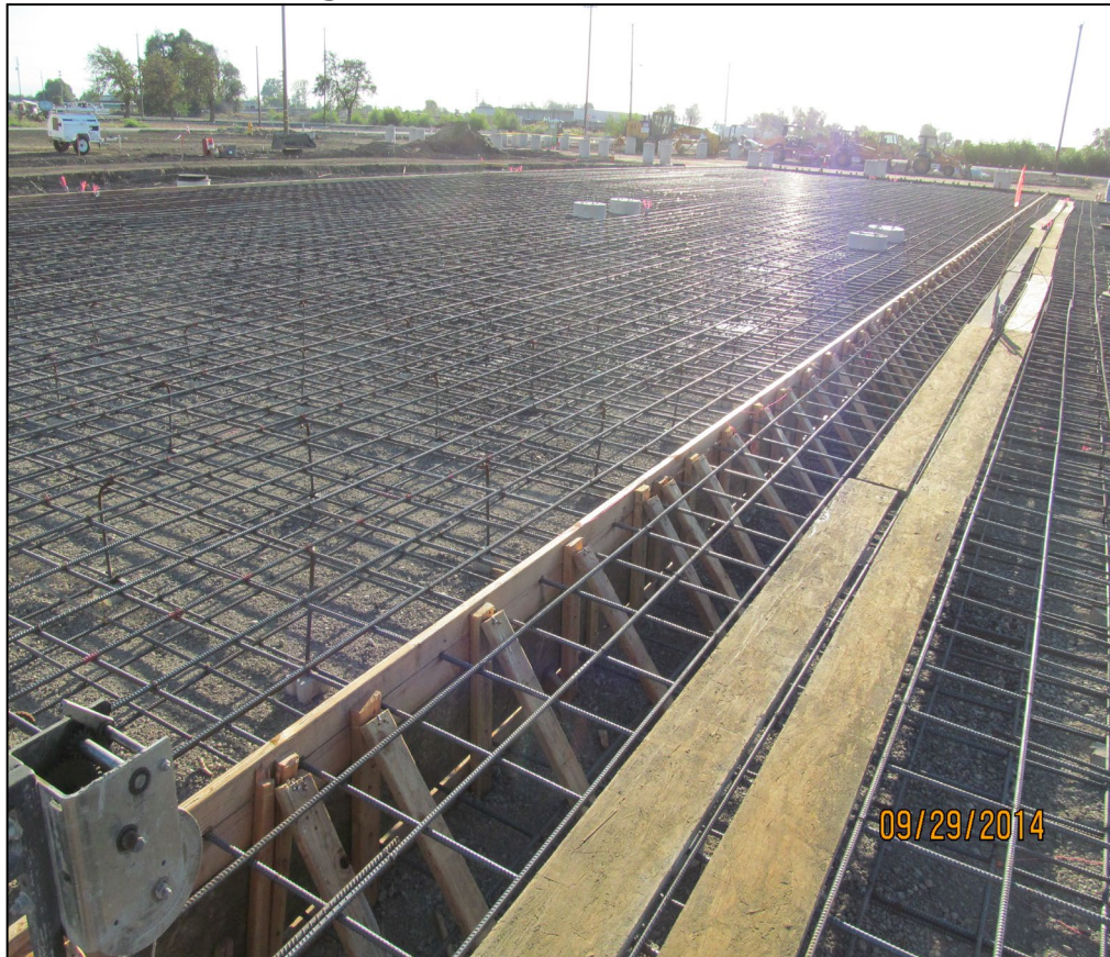
Figure 13: Rebar and Forms
