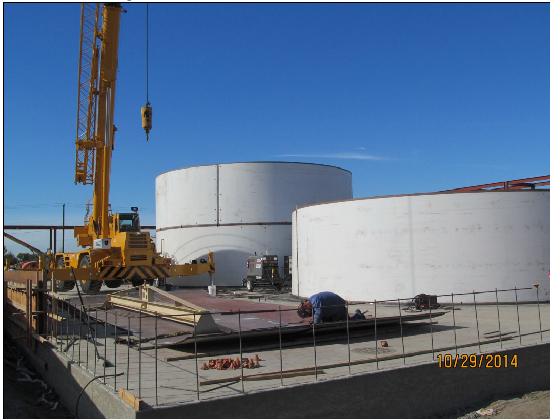
Figure 19: Second Level of Tank Erection
