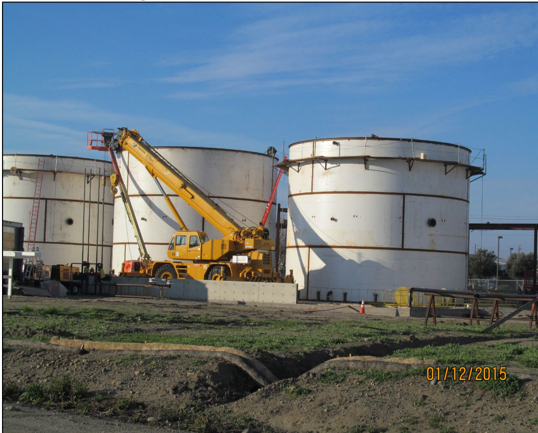
Figure 21: Third Level Tank Erection
