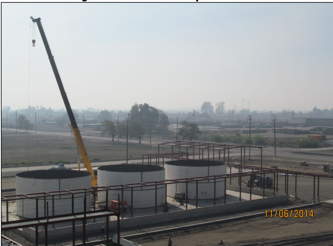
Figure 20: Tanks Partially Constructed
