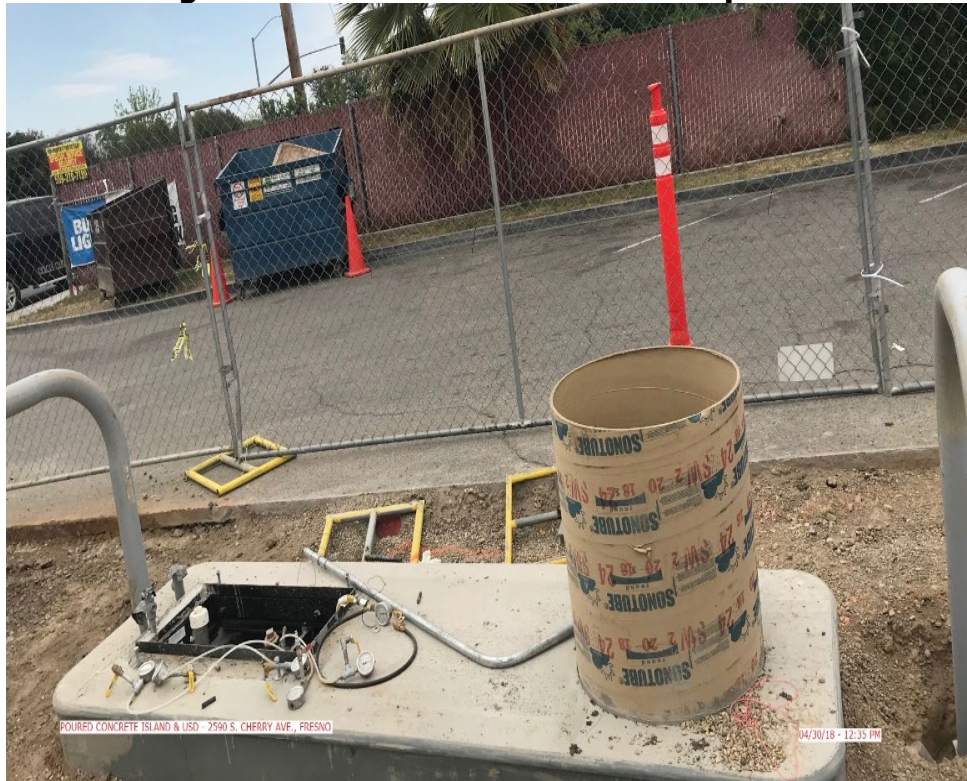
Figure 5: Concrete island for the dispenser
