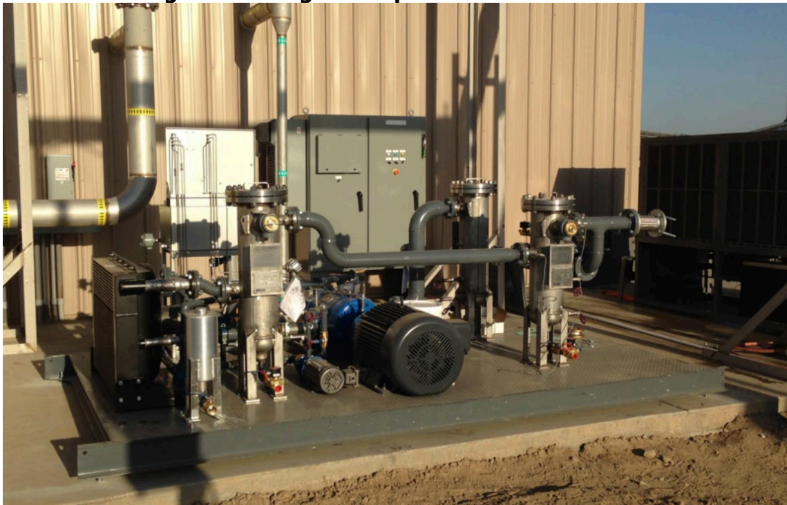
Figure 20: Biogas Compressor and Flowmeter
